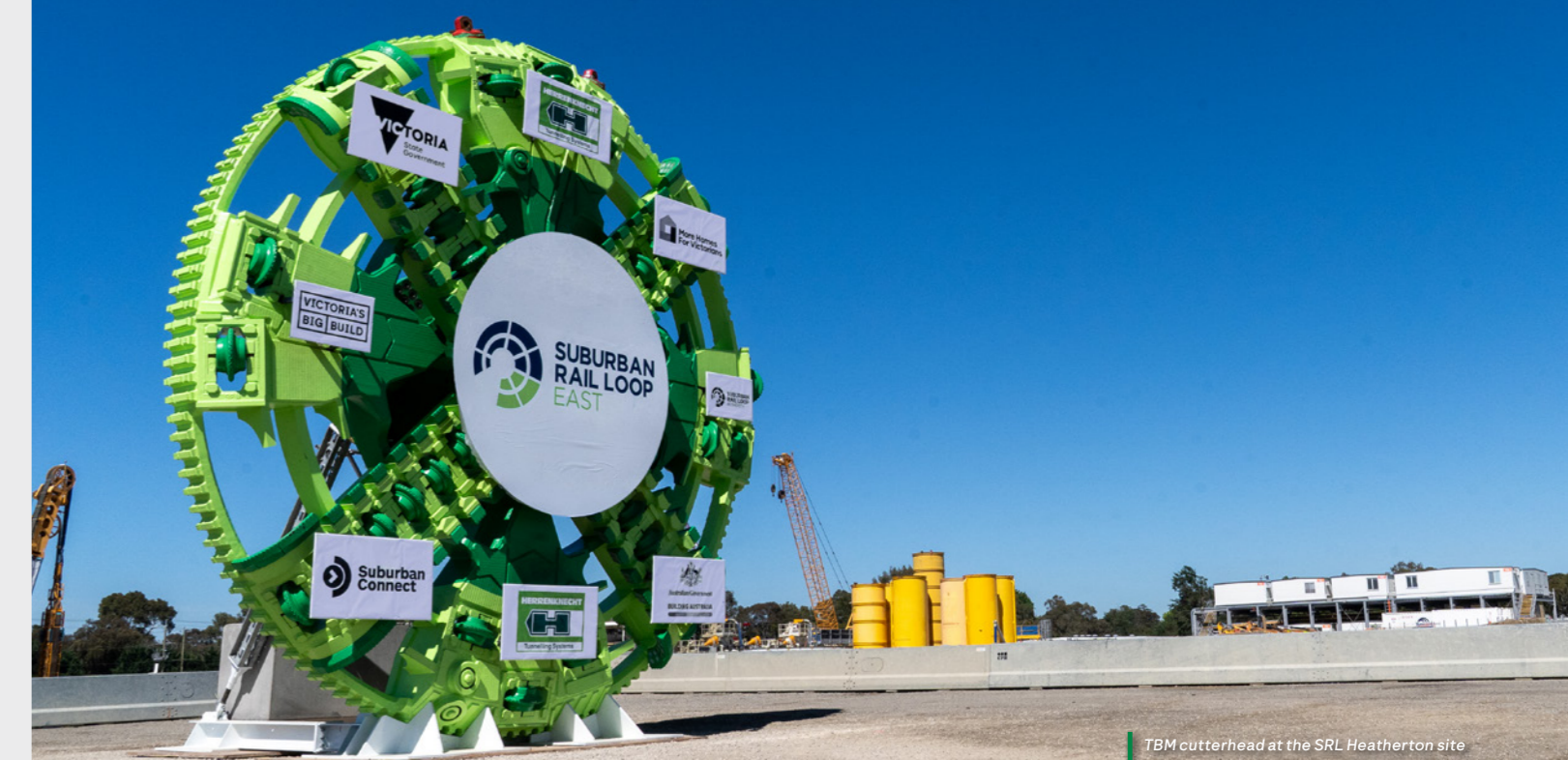
TBM cutterhead at the SRL Heatherton site
