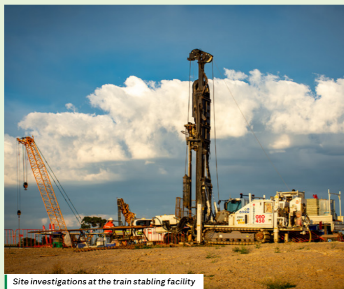
Site investigations at the train stabling facility
