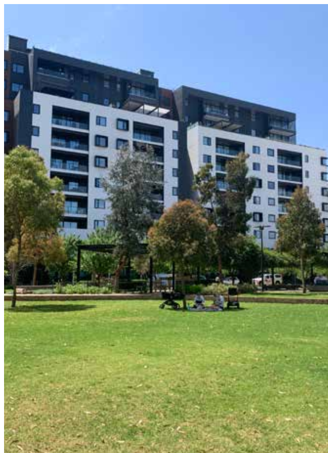
Apartment development located near open space
