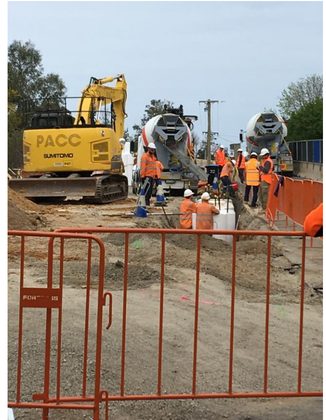
Guide wall works on Osborne Street, South Yarra
