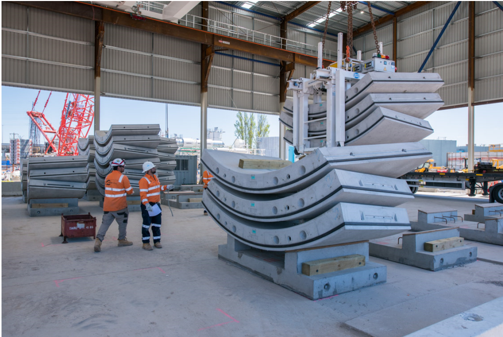
Pre-cast tunnel segments being delivered to site
