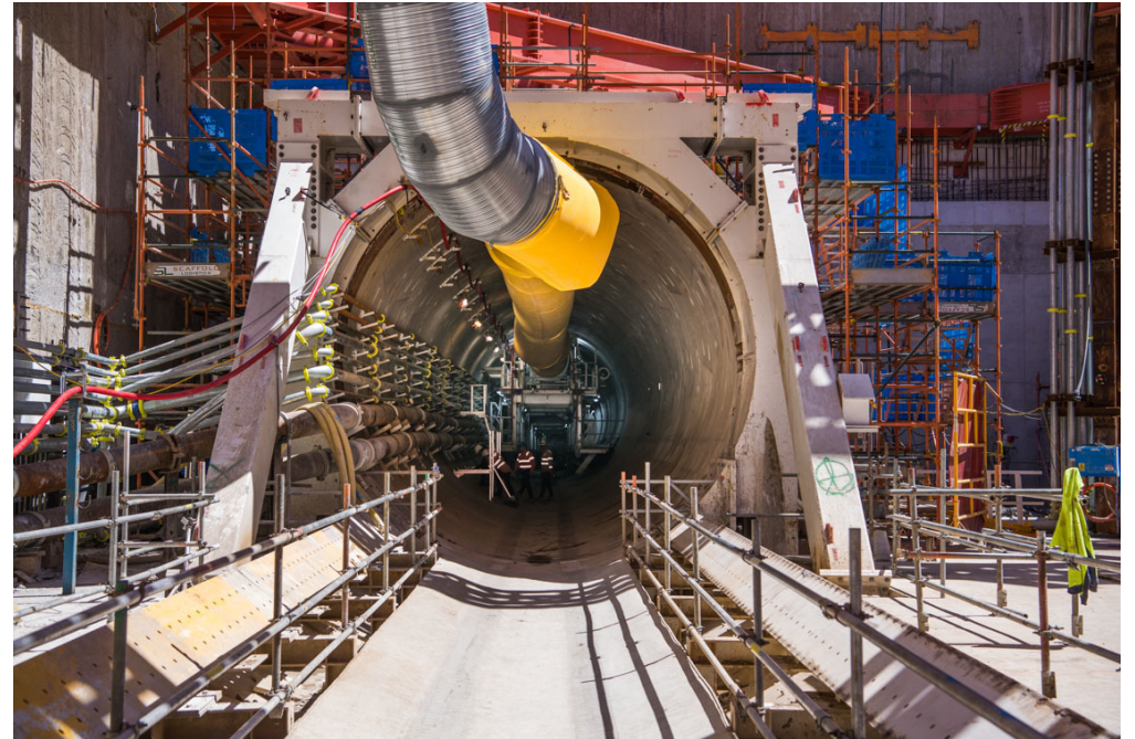
Looking into the first tunnel entrance via the steel bell
