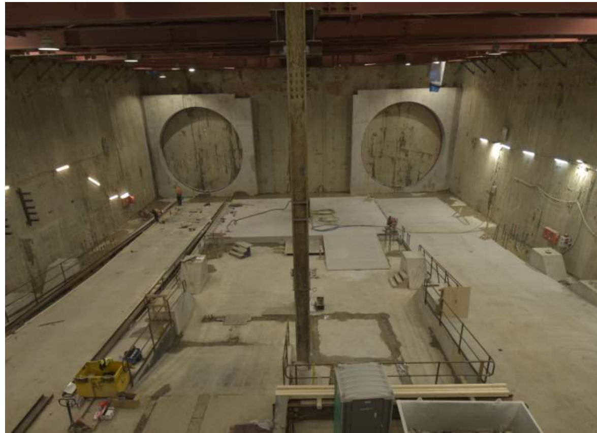
The northern end of the Anzac Station box
