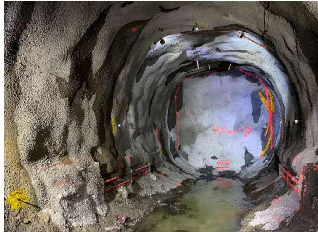
Cross Passage 2, between the Western Portal (Kensington) and Arden Station
