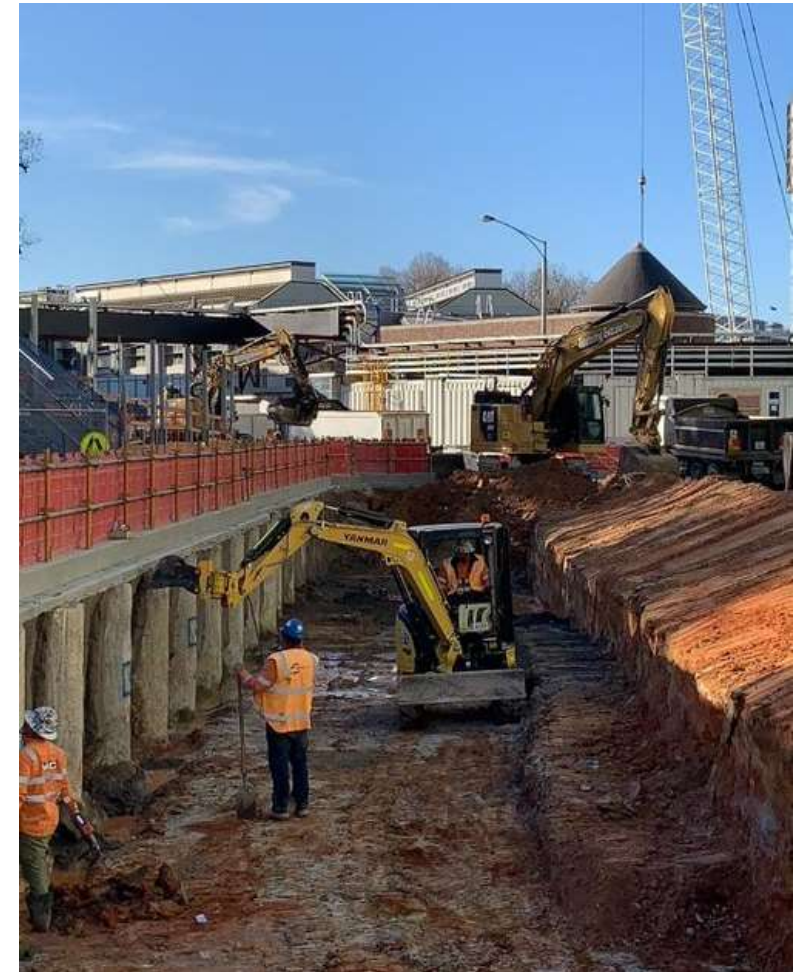
Excavation underway at the station entrance
