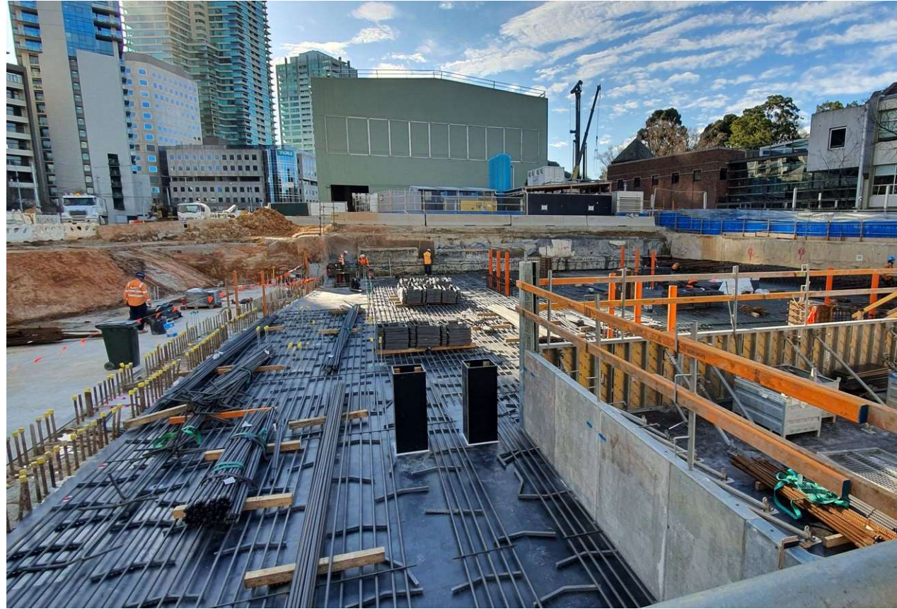
Steel reinforcements being installed ahead of the roof slab pour
