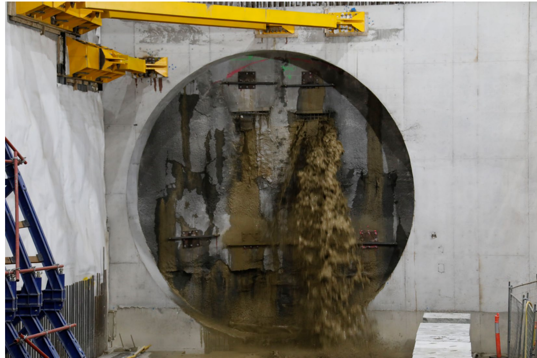
TBM Meg break through at Parkville – 19 September 2020
