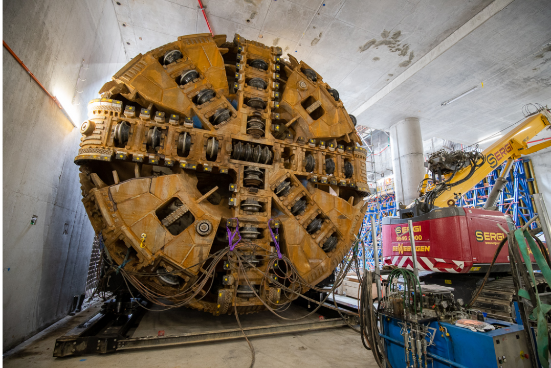
TBM Meg being transferred through the Parkville Station box
