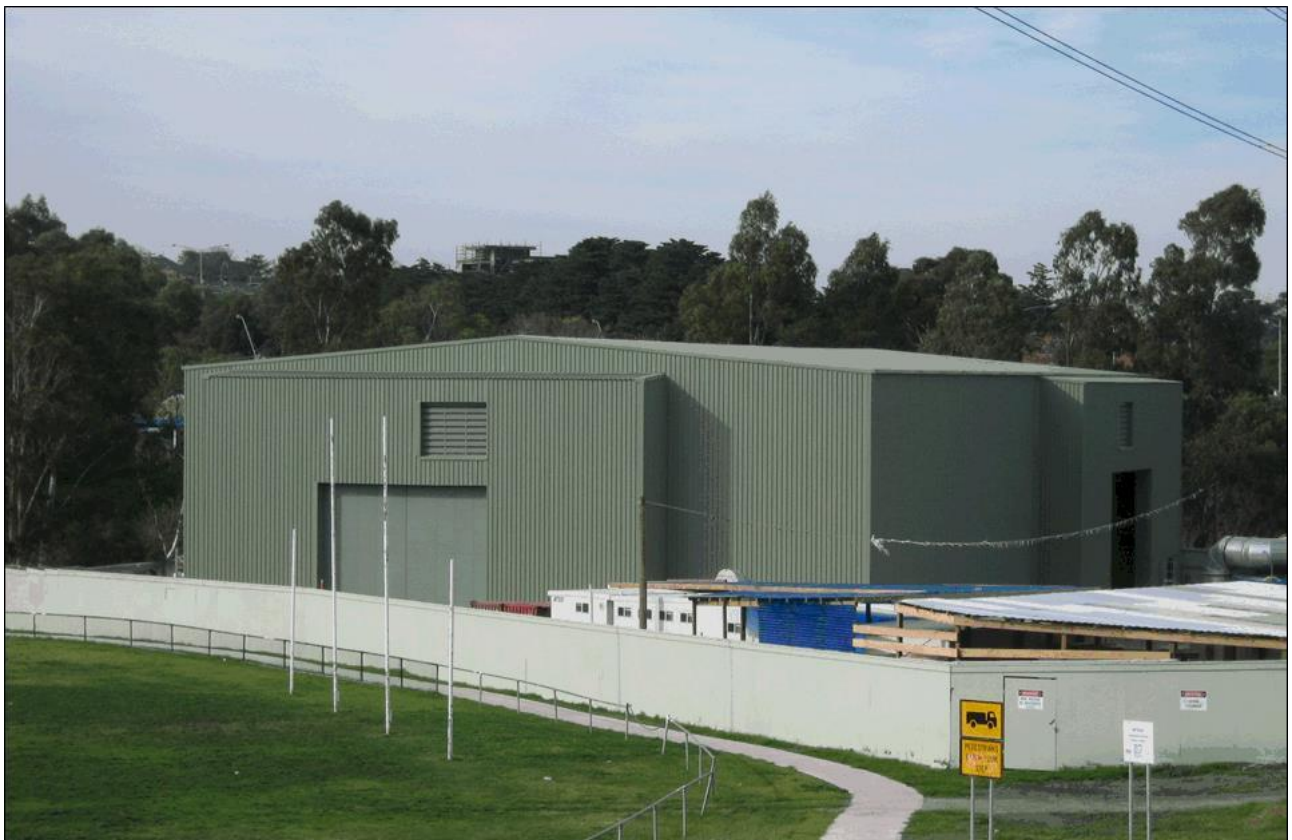
Figure 4-12: Acoustic Construction Shed
