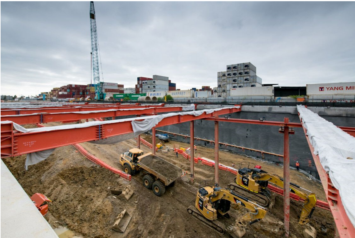
Photo 6 - North Portal bulk excavation and temporary support – Tunnel Zone (Source: WGTA, 19 February 2019)
