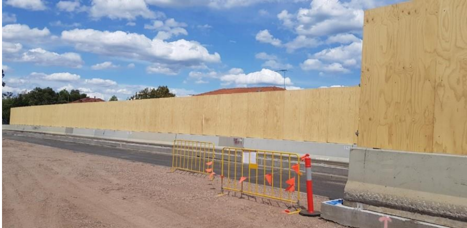
Temporary Noise Walls
