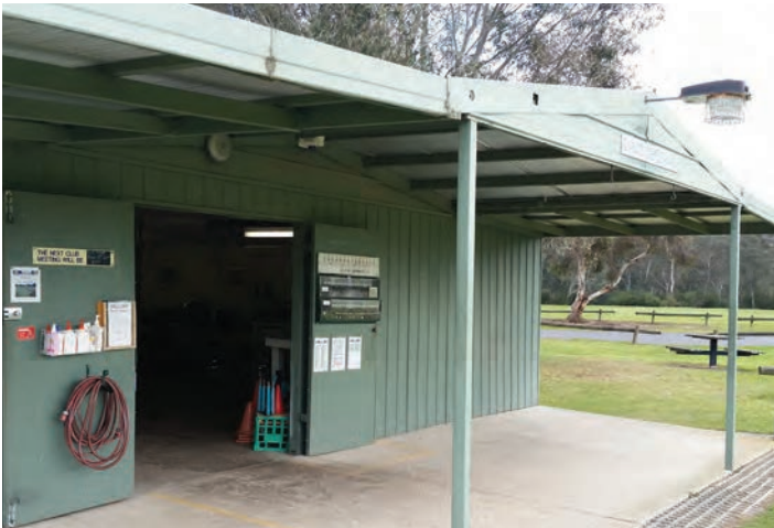
Figure B3.3 Existing aeromodelling facility in Bulleen Park
