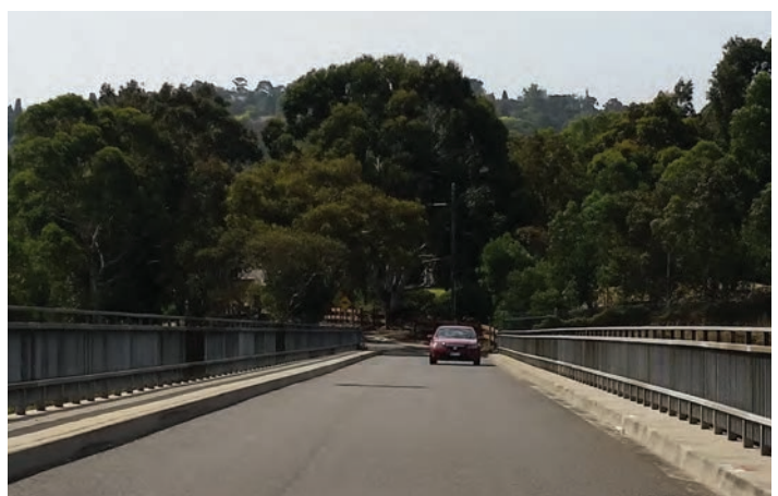
Figure 3.5 Vehicle bridge over Eastern Freeway providing access to Freeway Public Golf Course
