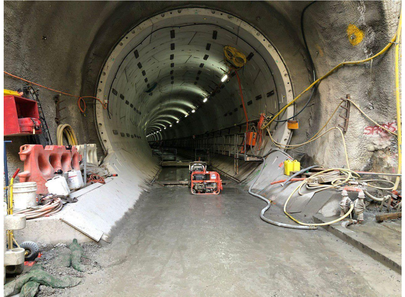
Eastbound tunnel invert complete
