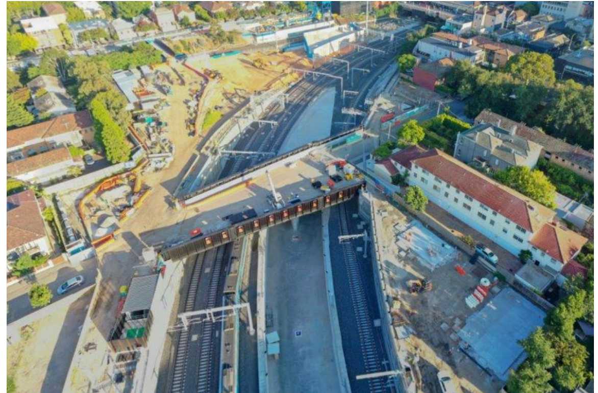
William Street Bridge access to decline structure
