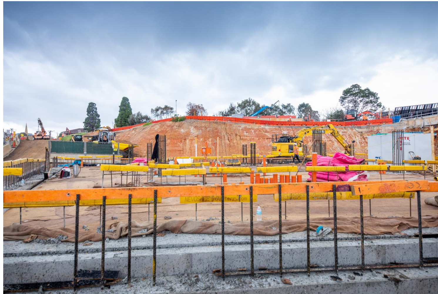
South Yarra substation works area
