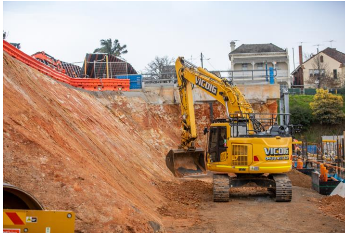
Siding Reserve works area
