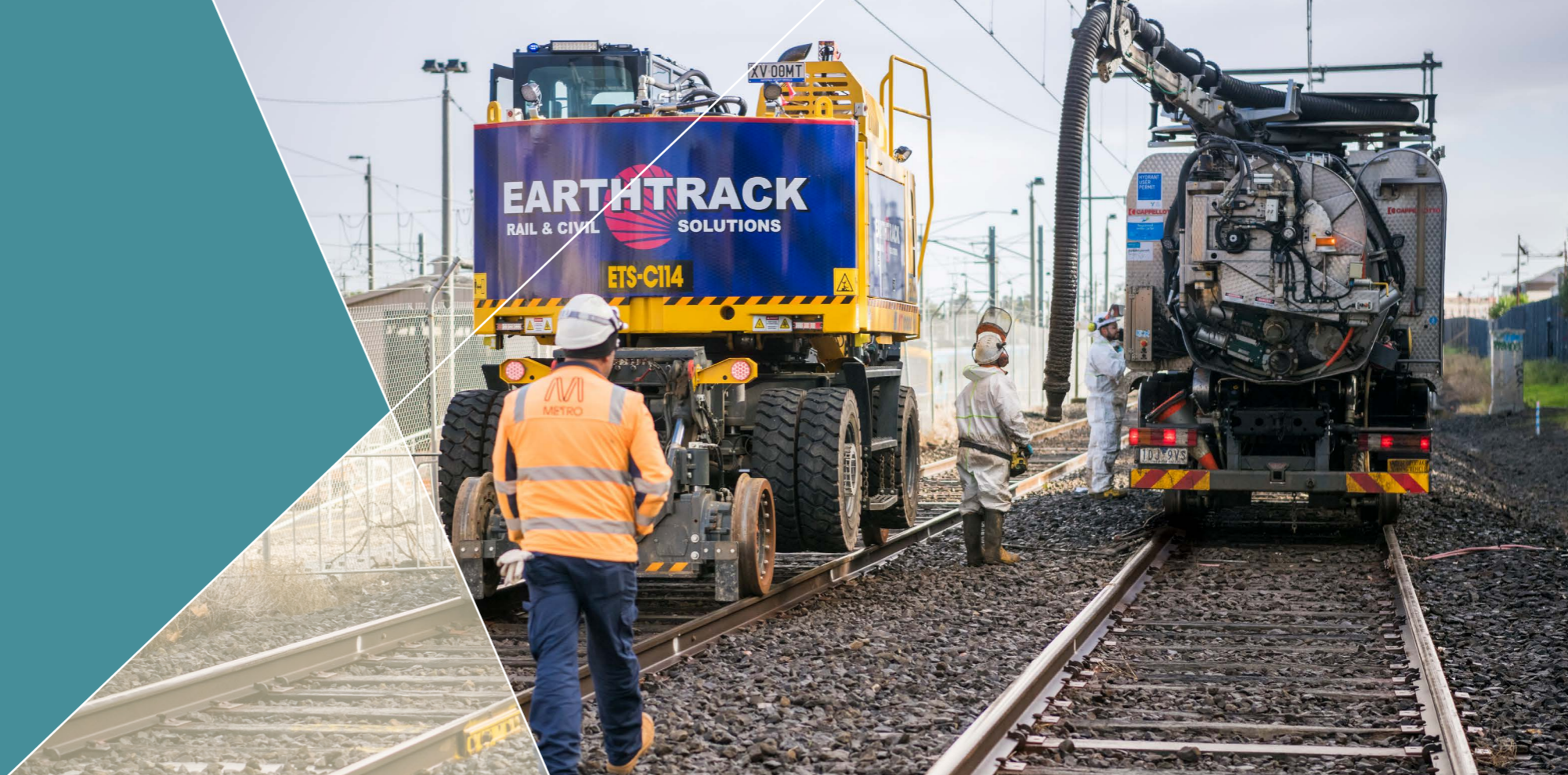
Working along the rail corridor
