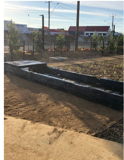
Figure 28. Timber culvert Reservoir station
