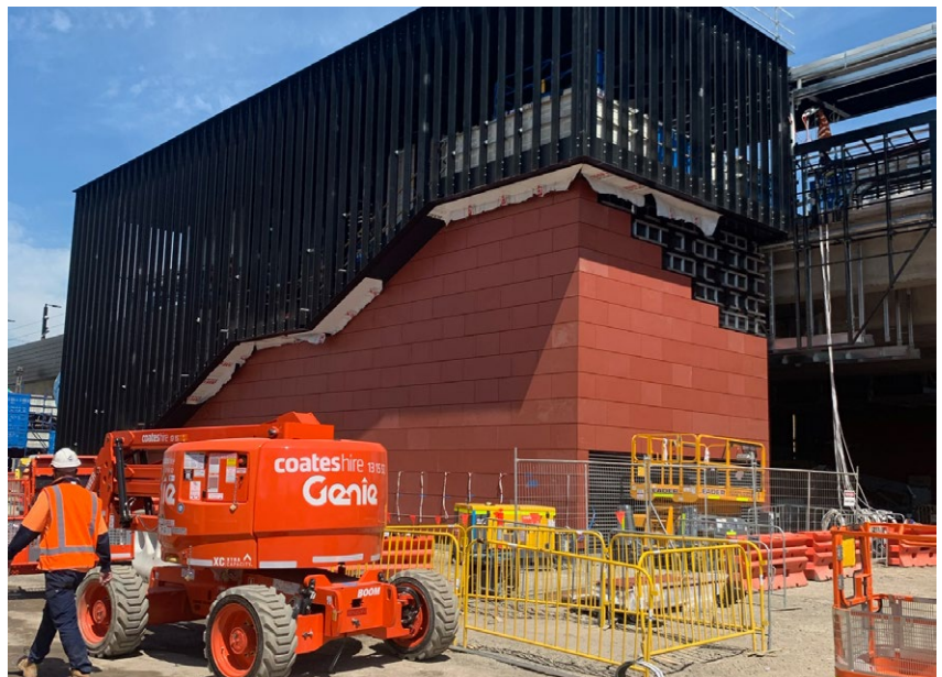
Figure 31. Moreland station facade references flemish bond brickwork of original station
