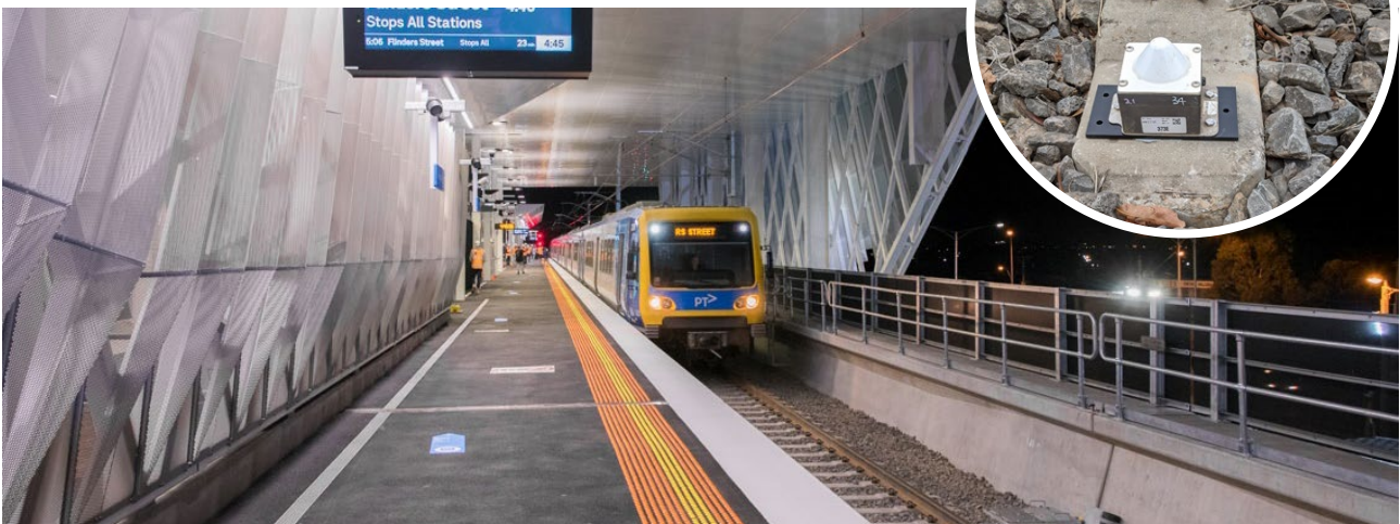
Figure 52. Tilt meters at Reservoir station
