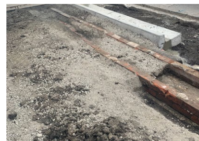
Figure 35. Drainage channel uncovered during subgrade preparation for permanent pedestrian path construction
