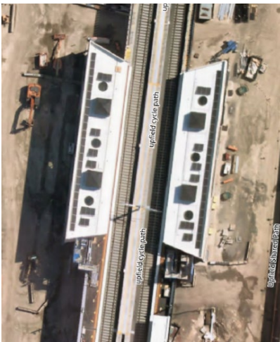
Figure 54. Solar panels at Moreland Station
