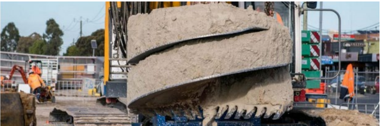
Figure 57. Monopiling at Reservoir station
