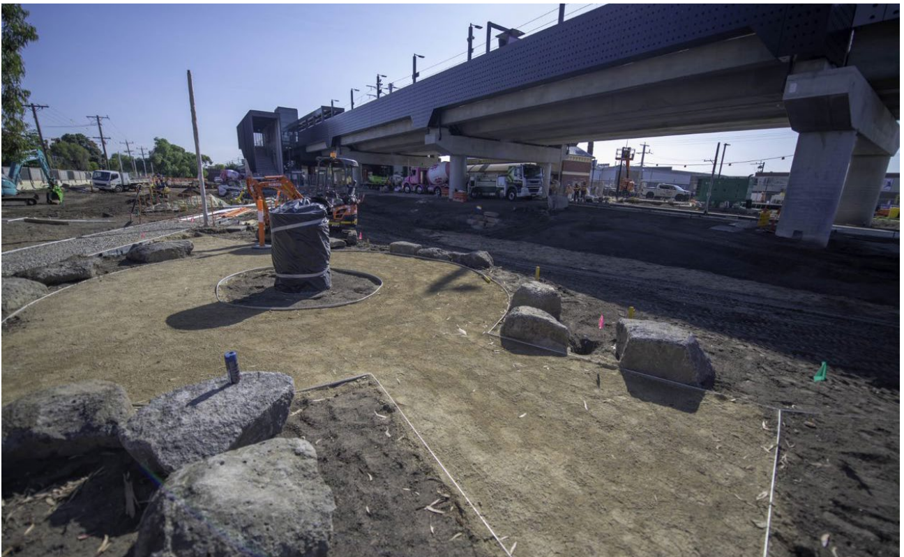
Figure 27. Canoe Tree and Yarning Circle at Moreland station under construction
