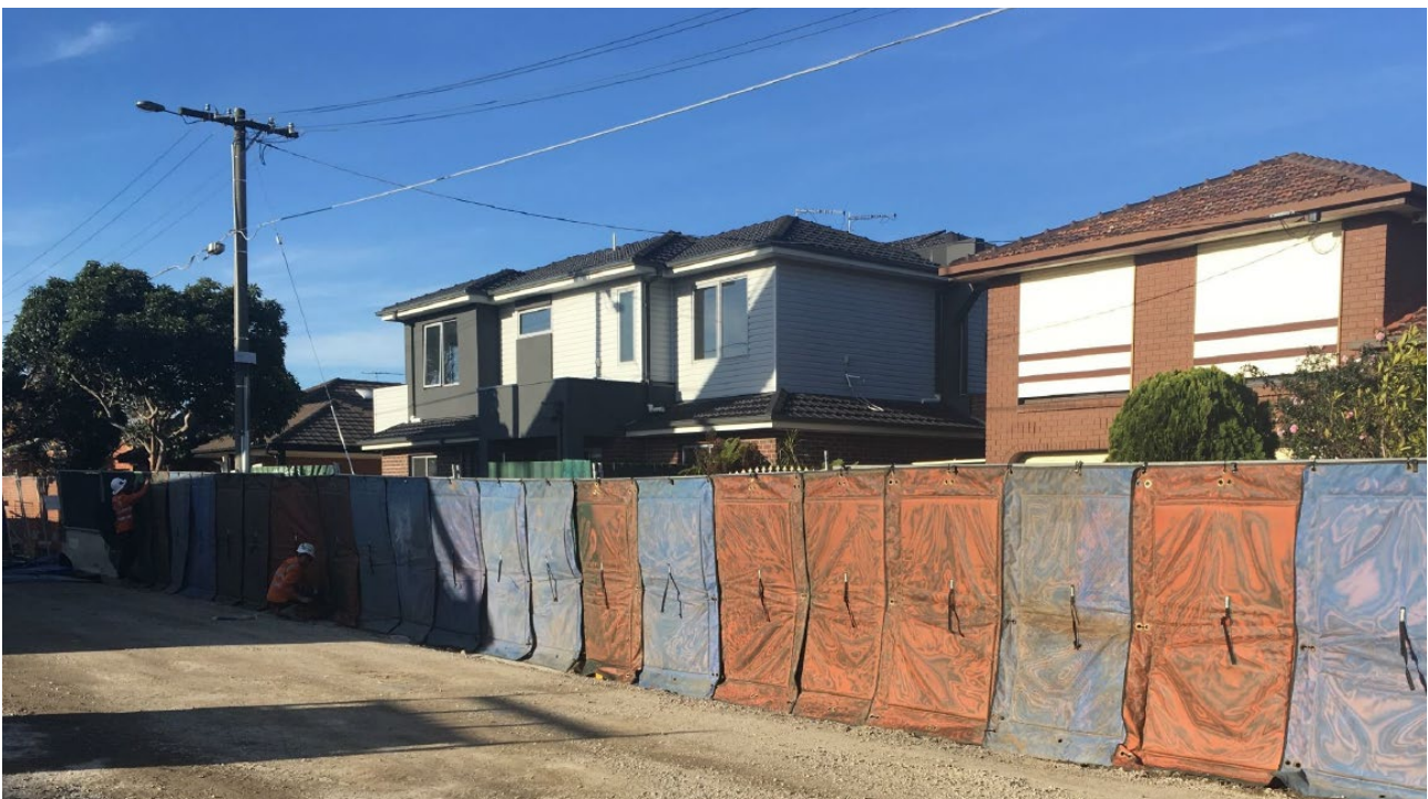
Figure 11. Macartney St, Reservoir during rail and retaining wall installation works
