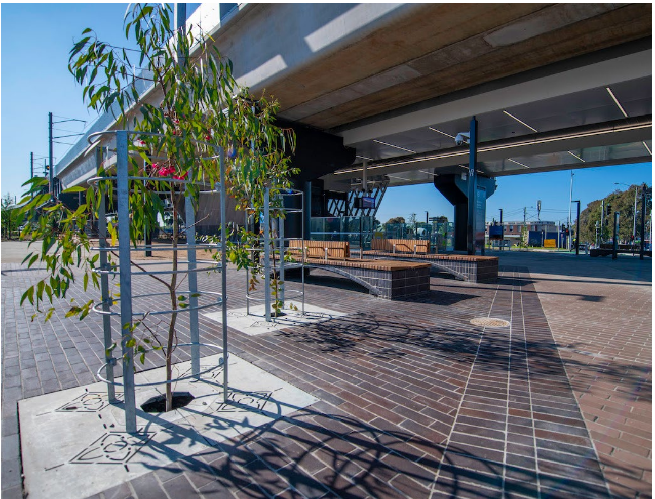
Figure 18. Landscaping establishment at Reservoir station
