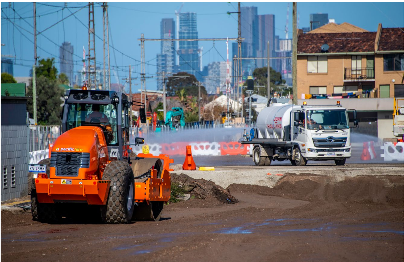
Figure 15. Dust suppression at Coburg station
