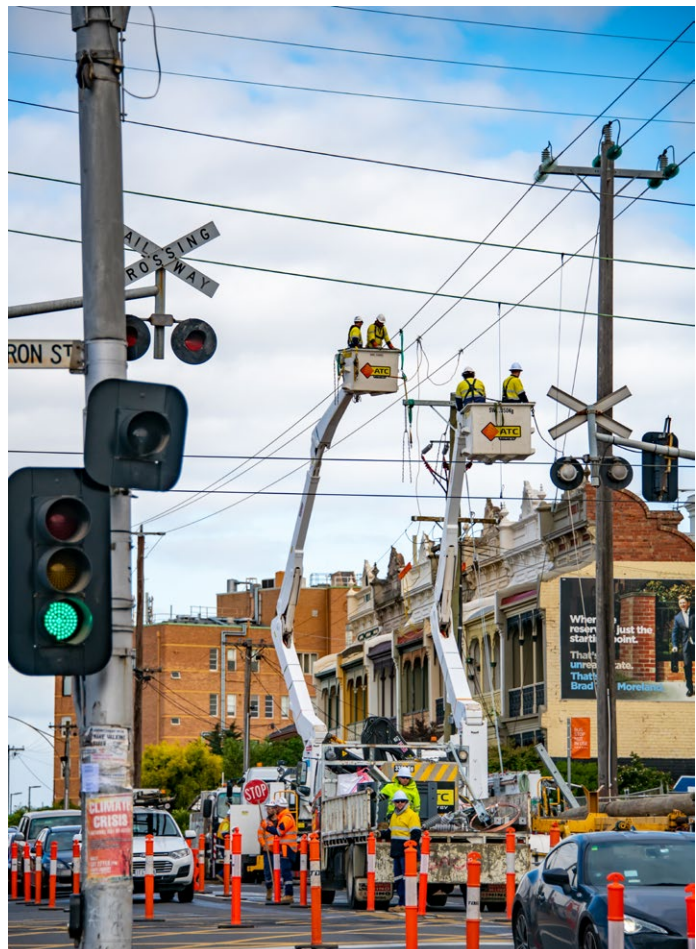
Figure 1. Overhead wiring works Bell to Moreland
