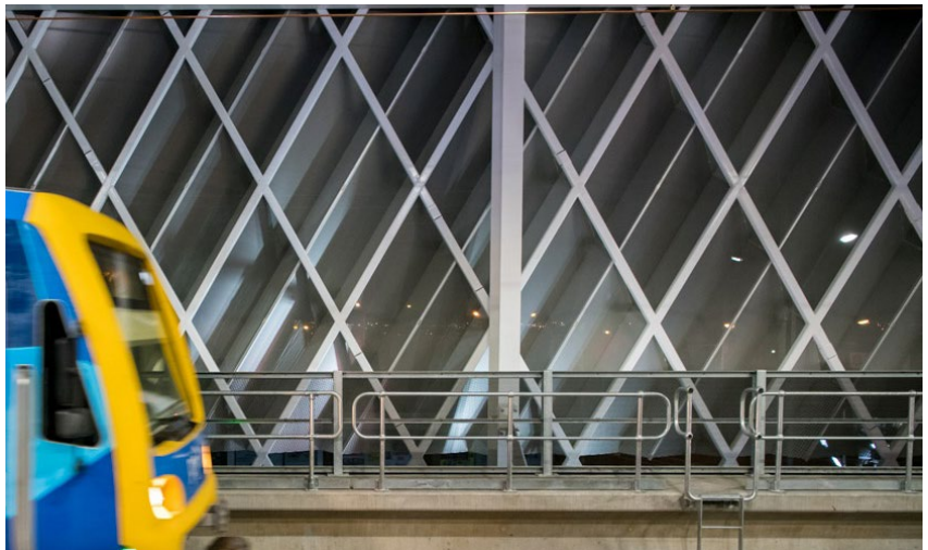
Figure 39. Aluminium screen at Reservoir station
