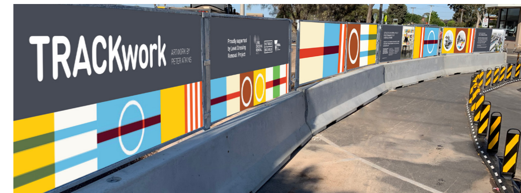
TRACKwork featured on the Hoppers Junction temporary pedestrian crossing
