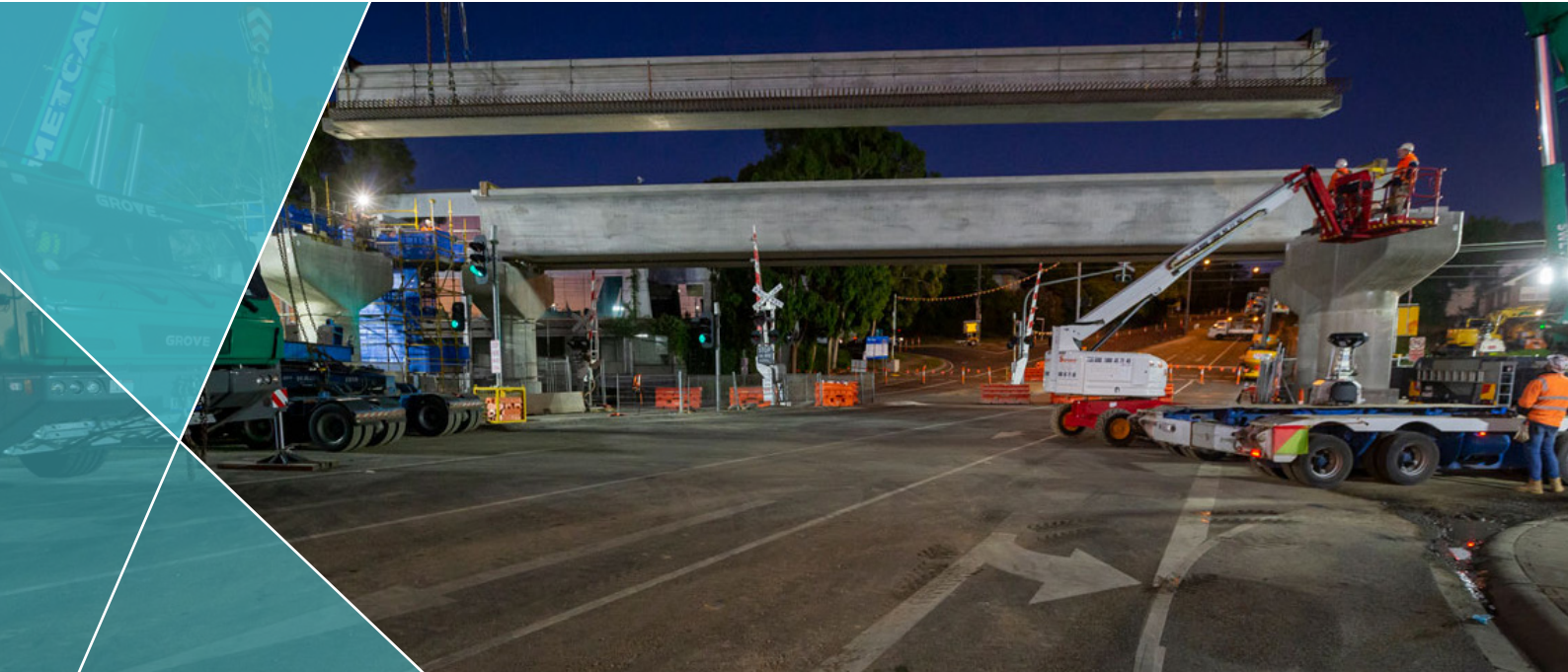
Beams being lifted for the rail bridge at Toorak Road
