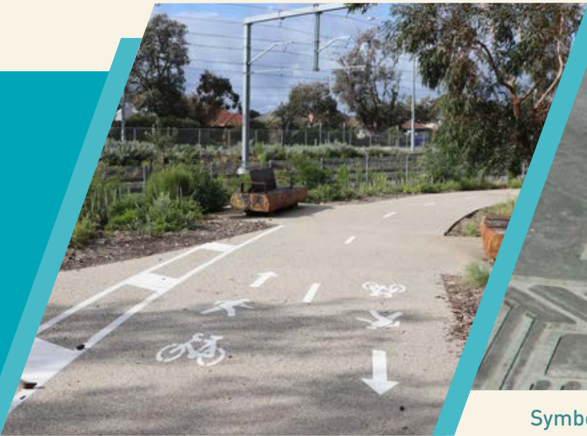
Completed section of the share use path in Seaford
