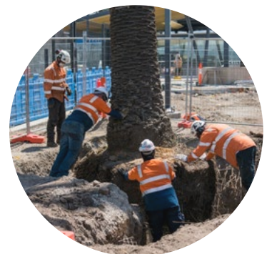
Construction workers position a returned date palm in Cheltenham
