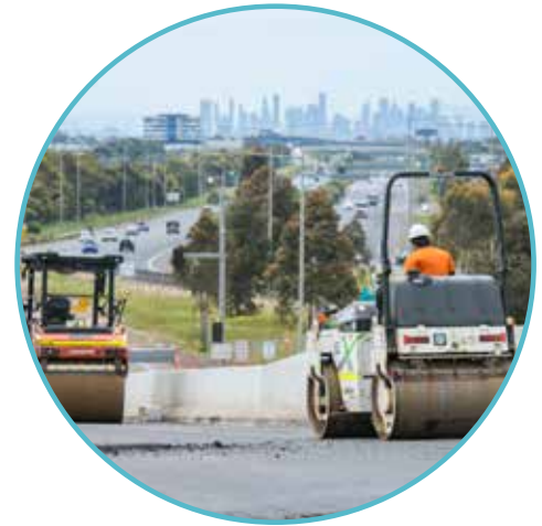
New road bridge off ramp, heading towards the city
