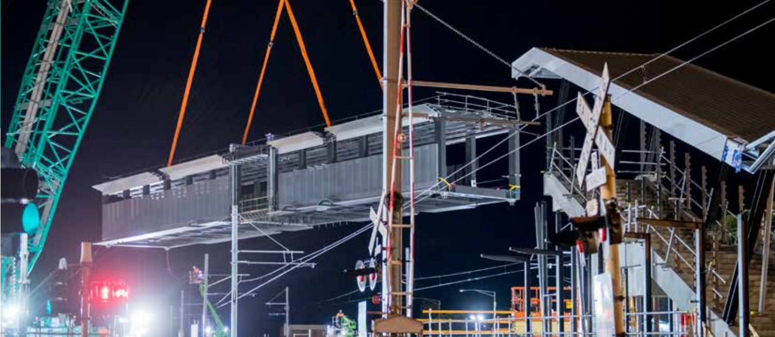
New pedestrian and cyclist bridge being lifted into place
