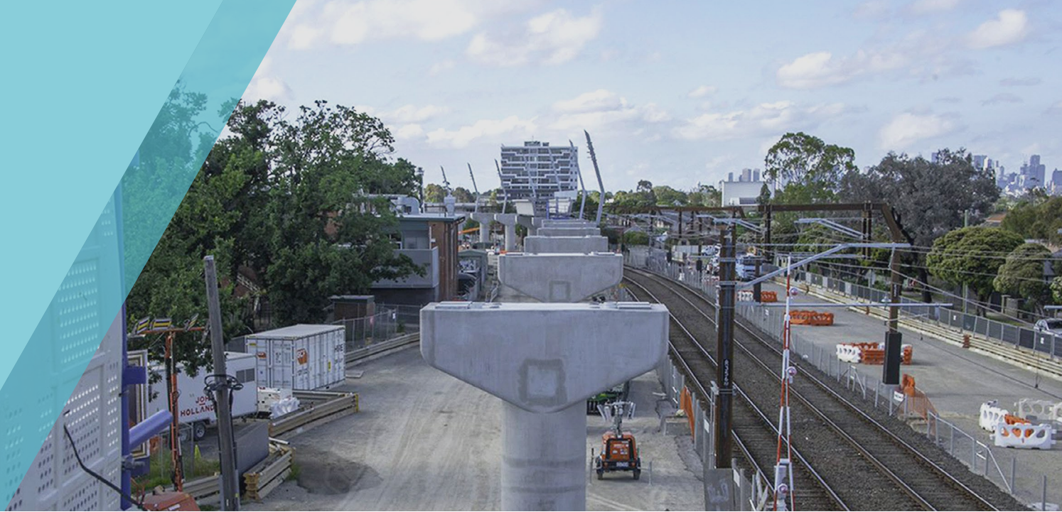
Piers and crossheads at Preston City Oval
