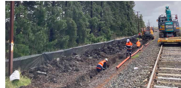
Figure 2: 1.2km of GGF fencing was placed along the work site.
