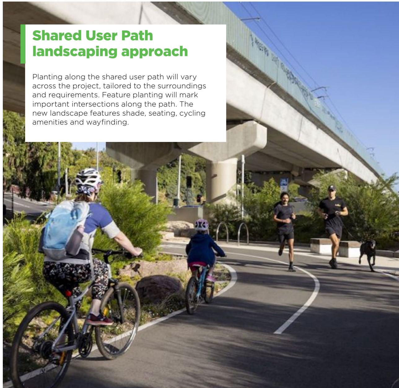
Example of landscaped shared user path (image of the Toorak Road level crossing removal and shared user path https://bigbuild.vic.gov.au/projects/level-crossing-removal-project/projects/toorak-road-kooyong )
