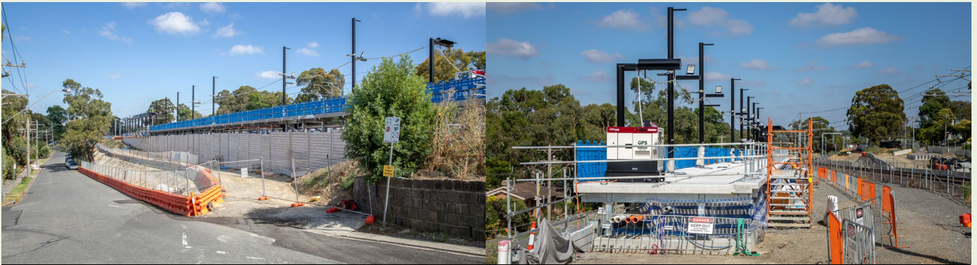
Two platforms being constructed at the new Montmorency Station
