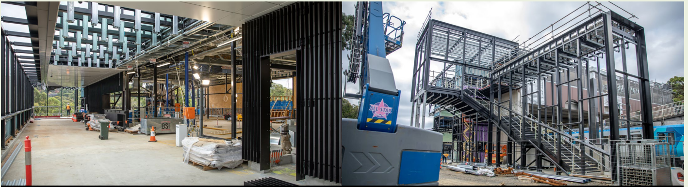
Works underway at the new Greensborough Station
