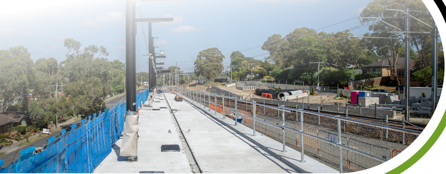
Structural works on the new Montmorency Station
