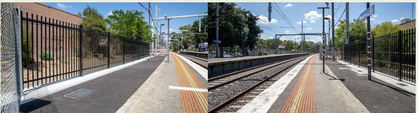
Platform 2 extension at Diamond Creek Station
