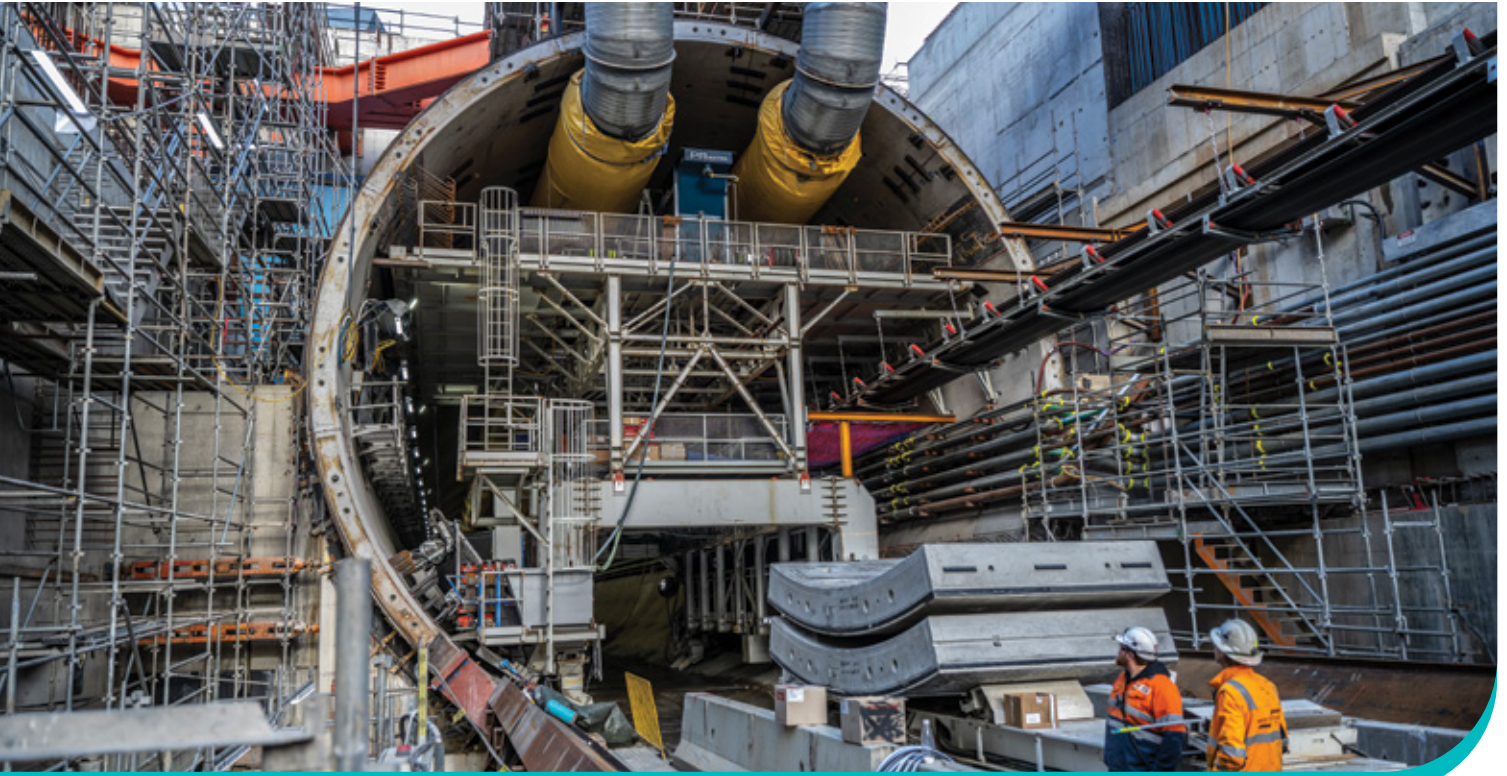
Exit of the citybound tunnel
