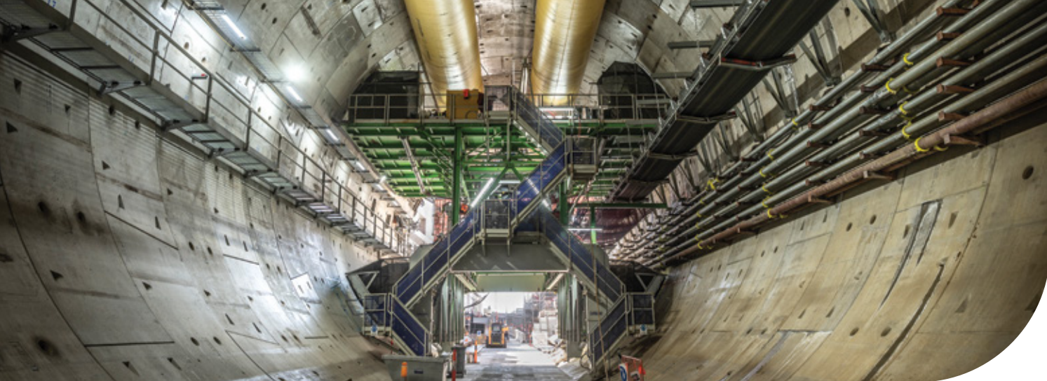
Back end gantries building the tunnels
