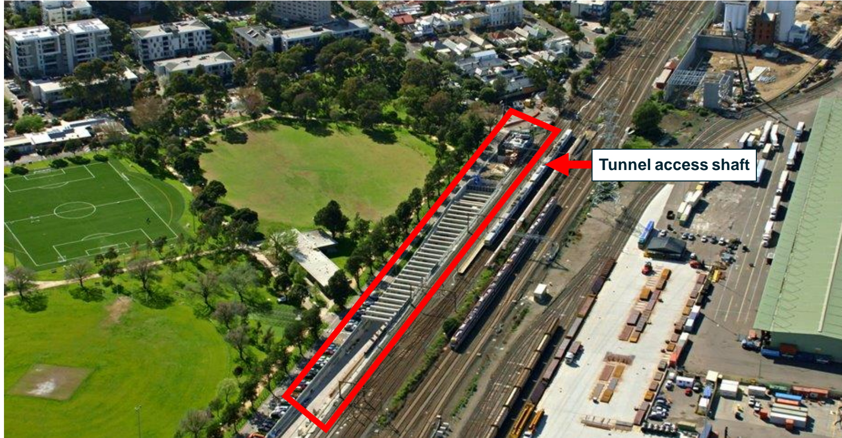
Image: The tunnel access shaft and western portal in South Kensington as part of Metro Tunnel Project.
