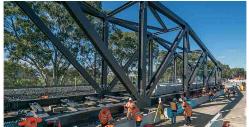
Eumemmerring Creek bridge construction
