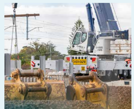
Machinery on the work site.
