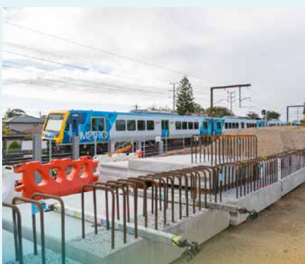
Train passing by the Parkdale worksite on the temporary track.
