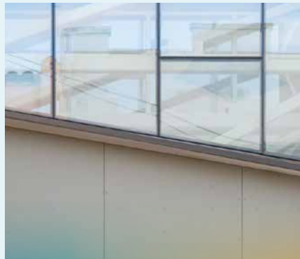
Close up of the glass panelling on the lift shaft.
