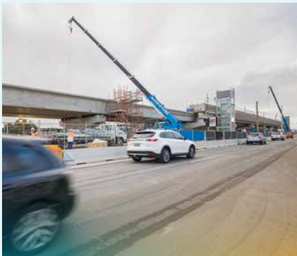
The new rail bridge taking shape over the rail line.
