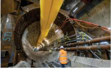
Hydraulic jacks push the TBM forward. As it moves forward, thick segments of pre-cast concrete are progressively installed behind the cutterheads. These concrete segments form a reinforced ring and are designed to fit together to create a permanent lining for the tunnel.
