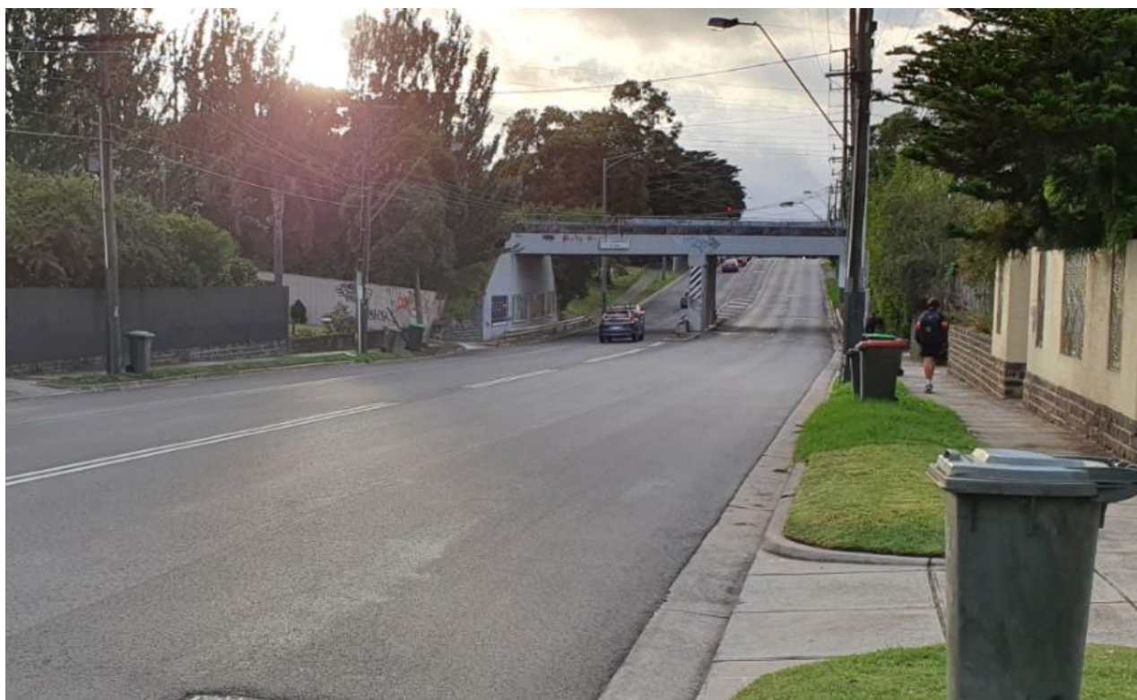
FIGURE 2.11 BAY ROAD UNDERPASS
