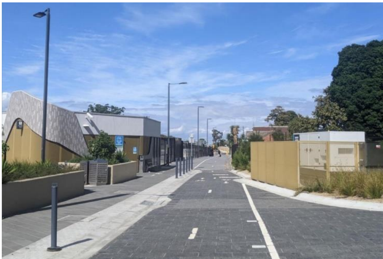
FIGURE 2.15 SHARED USE PATH AT CHELTENHAM STATION (SOURCE: SRLA 2022)
