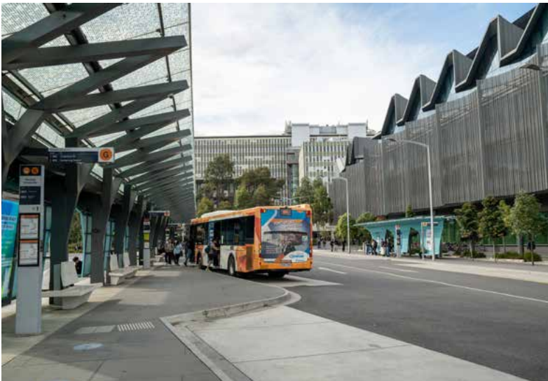
Monash University bus interchange
