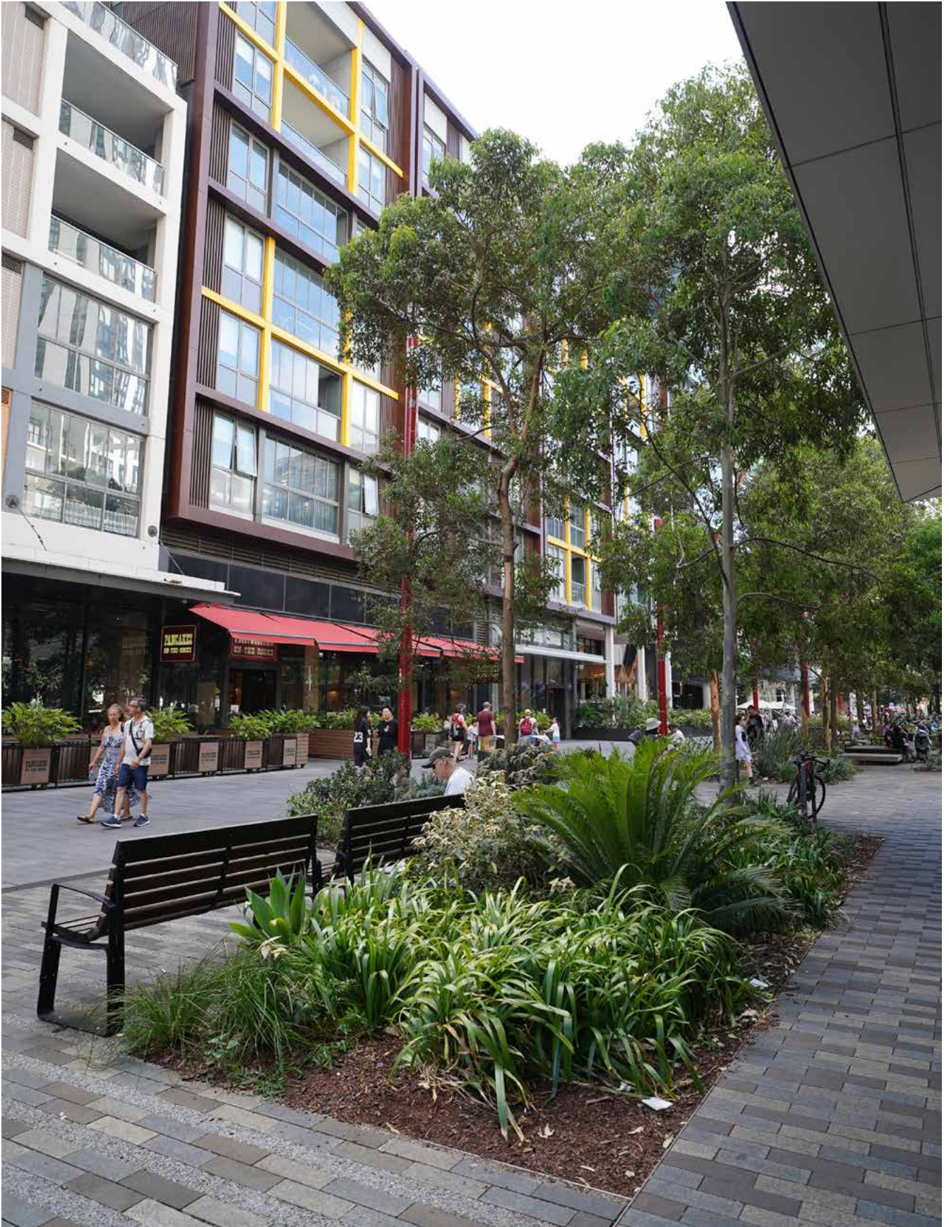
Urbanised street supporting public life. Darling Square, Sydney NSW
