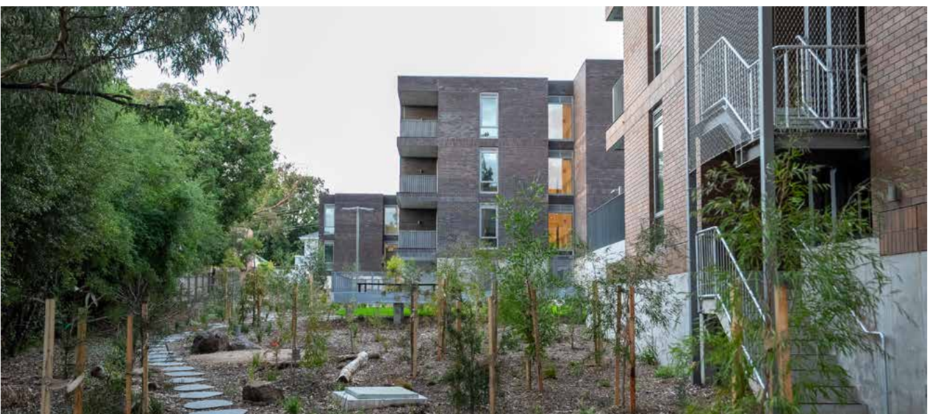
Social and affordable housing development at Markham Avenue Ashburton (supplied by Homes Victoria)
