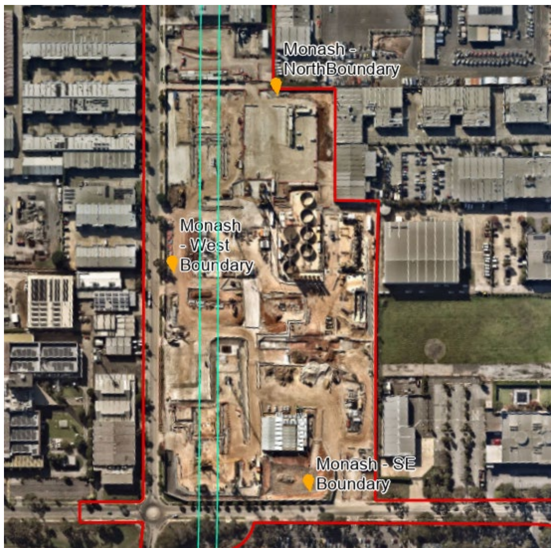
Figure 9: Monash air quality monitoring stations
