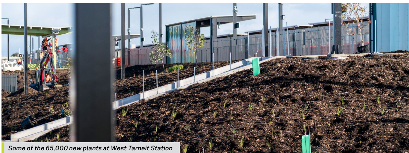
Planting underway at West Tarneit Station
