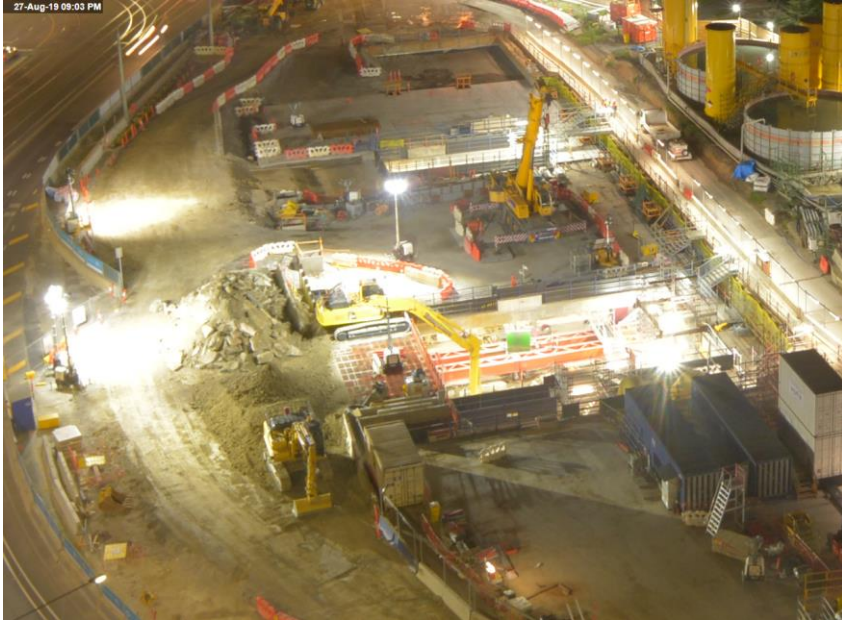
Lighting up to 10pm (excavation from surface)
