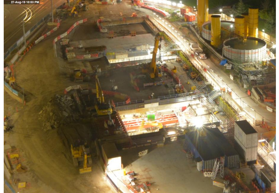
Lighting 10pm to midnight (excavation and strutting below ground)
