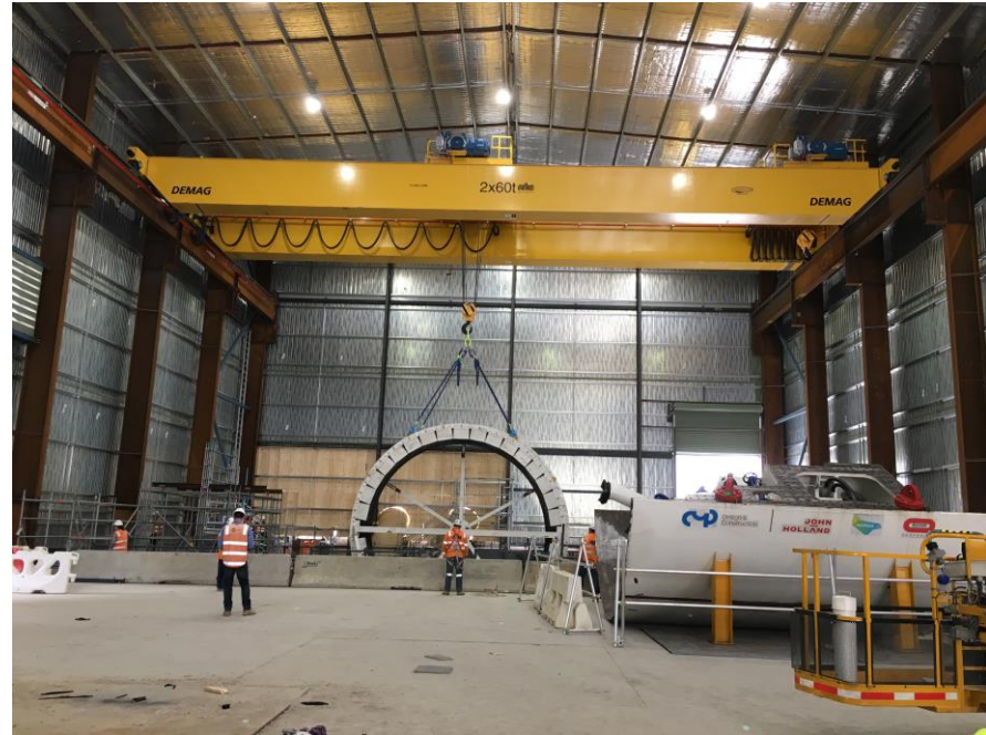
Launch ring lowering into Anzac Station
