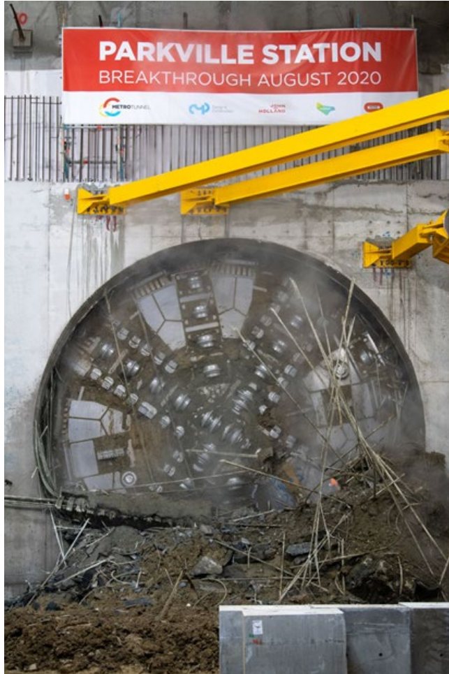
TBM Joan break through at Parkville – 27 August 2020
