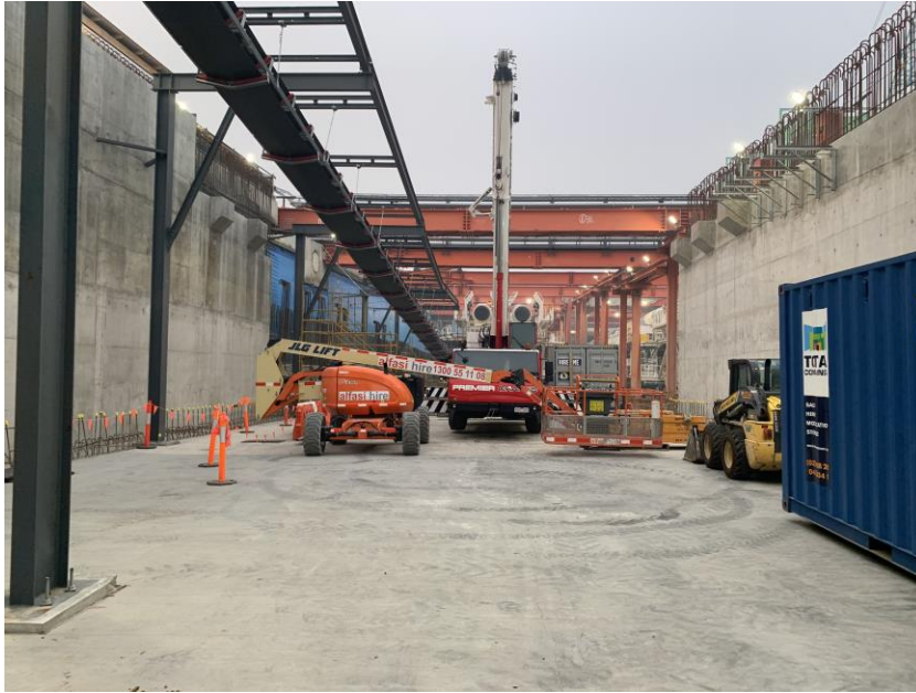
Wall and corbel construction
