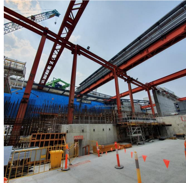
Maintenance level road deck
