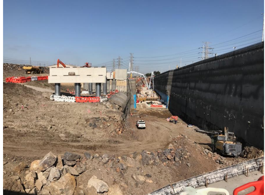
Cut and cover works at Outbound TBM retrieval pit
