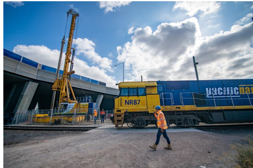
E Gate Site Establishment
