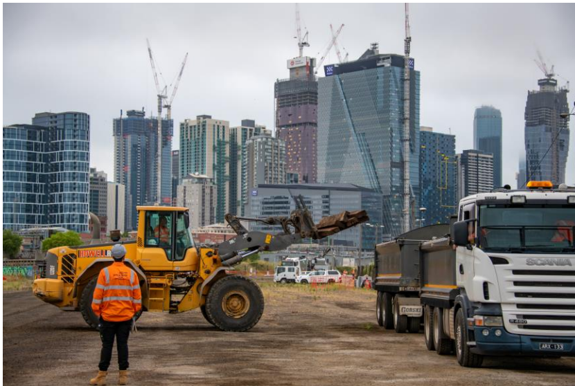
Appleton Dock Bored Piling
