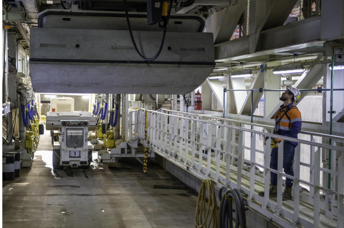
TBM tunnel ring crane
