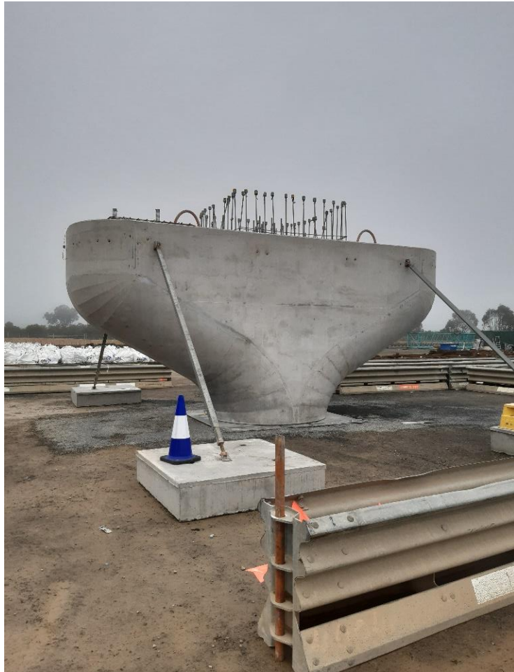
Concrete crosshead at Benalla
