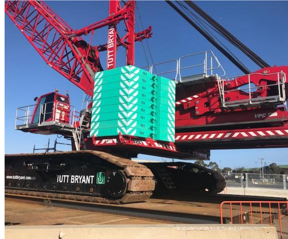
Works on CityLink structure
