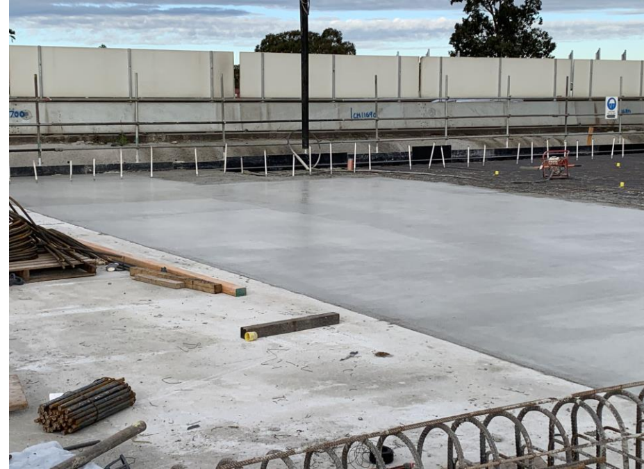
Building the new tunnel entrance roof
