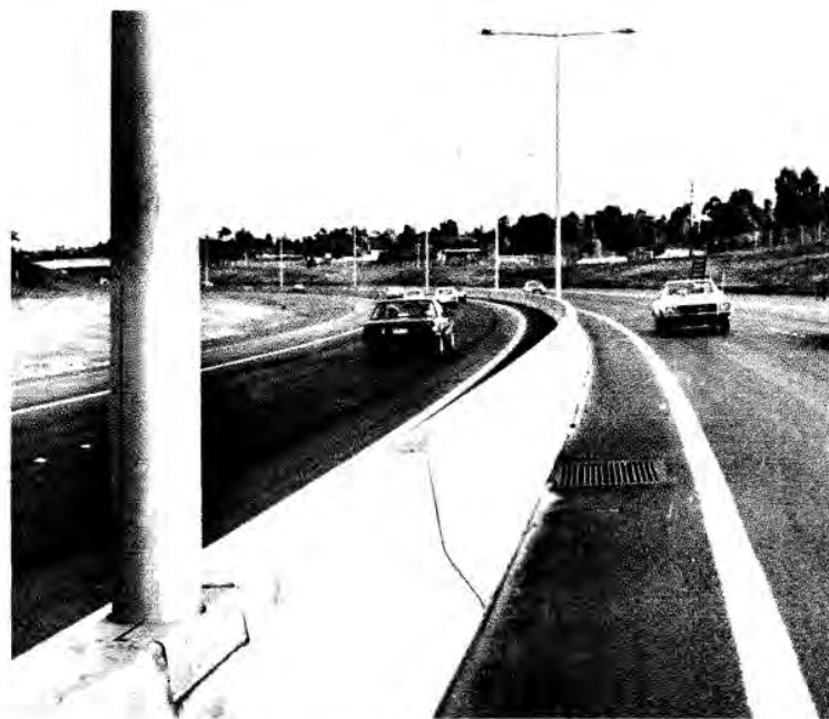
Figure C.54 New precast concrete median barriers in Bulleen-Doncaster extension of Eastern Freeway, 1982 (CRB, Annual Report, 1982)
