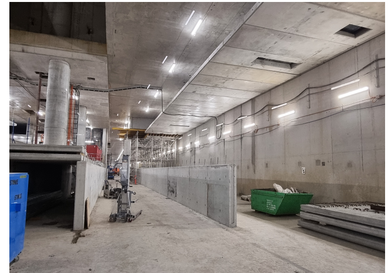
Over-track exhaust installation and platform wall construction
