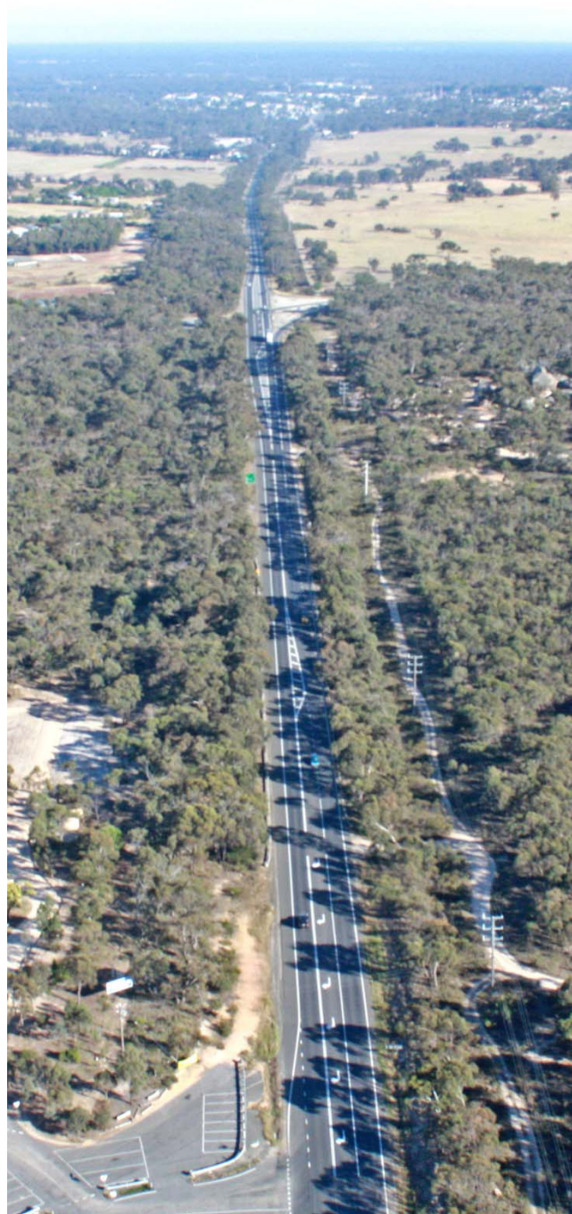
Western Highway looking north to Stawell from Panrock Reservoir Road intersection
