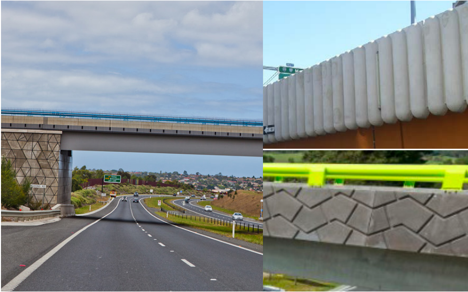
Architecturally designed bridge parapet
