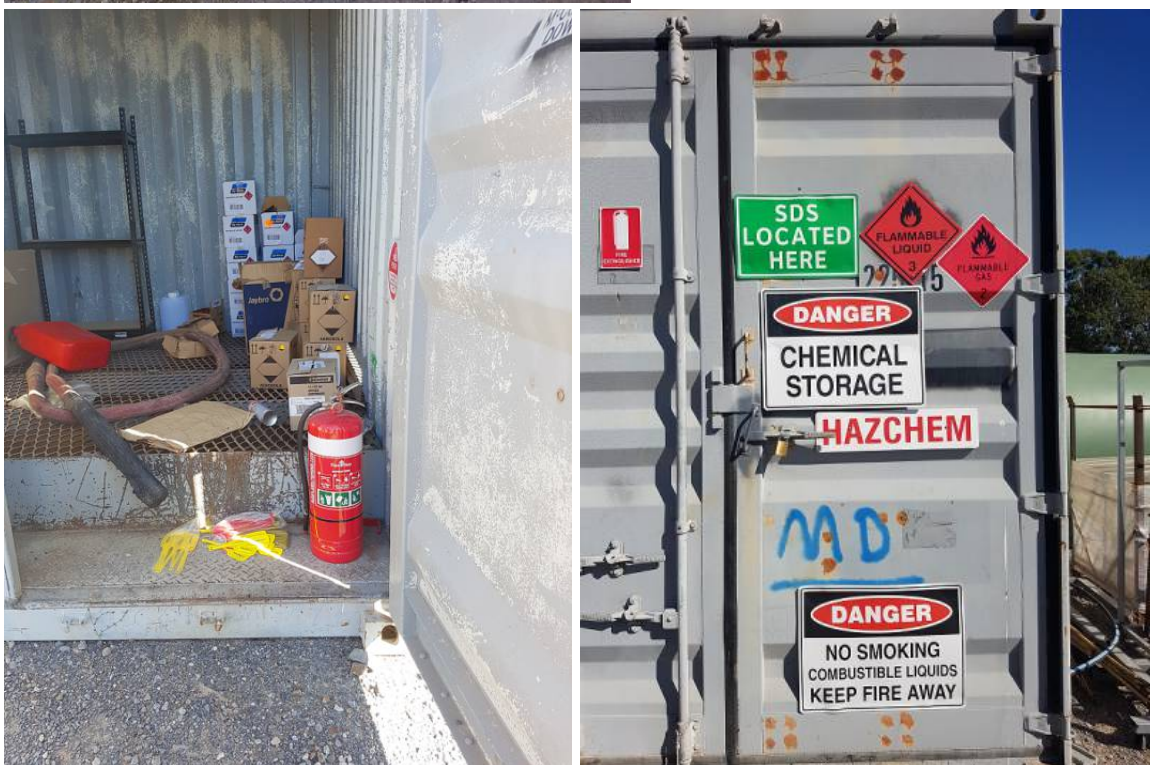
Left: Fire extinguisher inside the Dangerous Goods container at the Woodlands compound, making it impossible to retrieve in case of a fire in the container.
