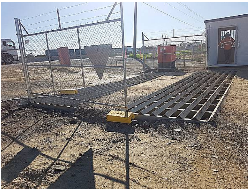
Left: Rumble Grid at exit of Governor Road compound.
