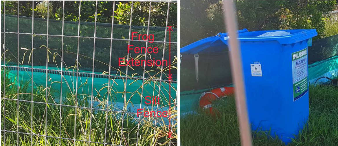
Left: Example of the combined sediment and frog fence south of Bowen Parkway Right: Marine spill kit in use around the waterways.
