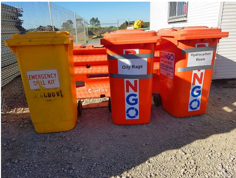
Above: A good example of well labelled and accessible waste bins and spill kits– Governor Road Compound.
