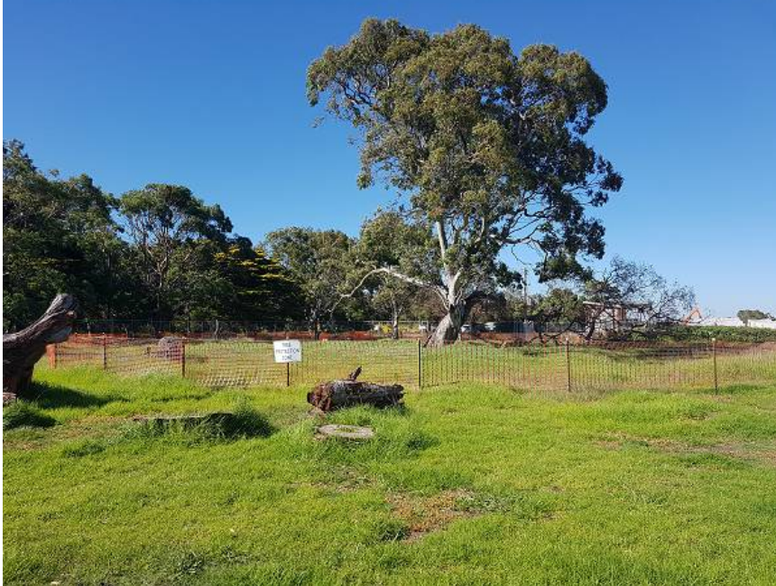
Left: Example of “No-Go” Zone fencing around a large gum tree west of the Parks Victoria compound.
