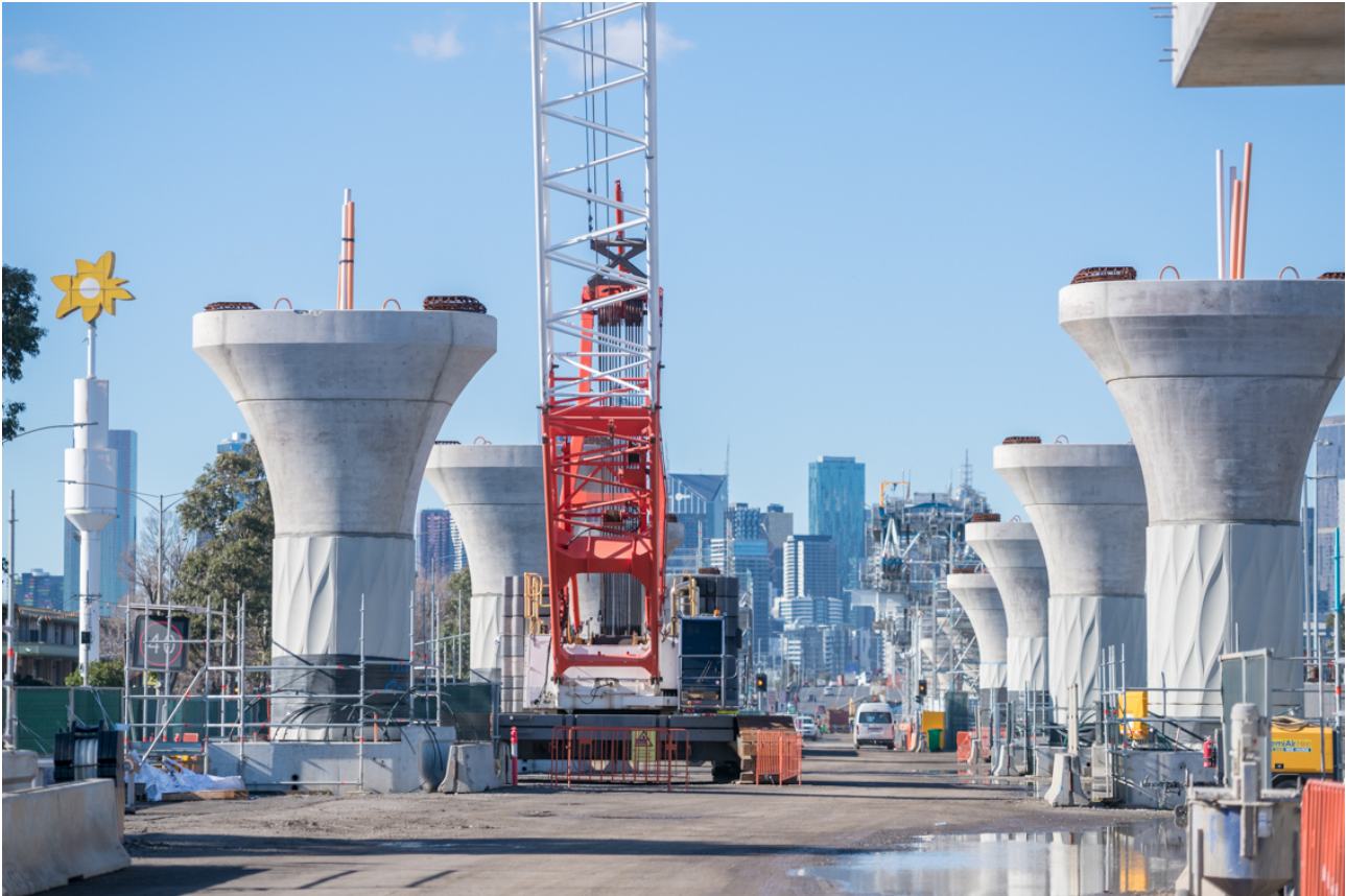
Photo 1 – Precast pier elements along Footscray Road – East Zone (Source: WGTP MTIA, 12 June 2021)
