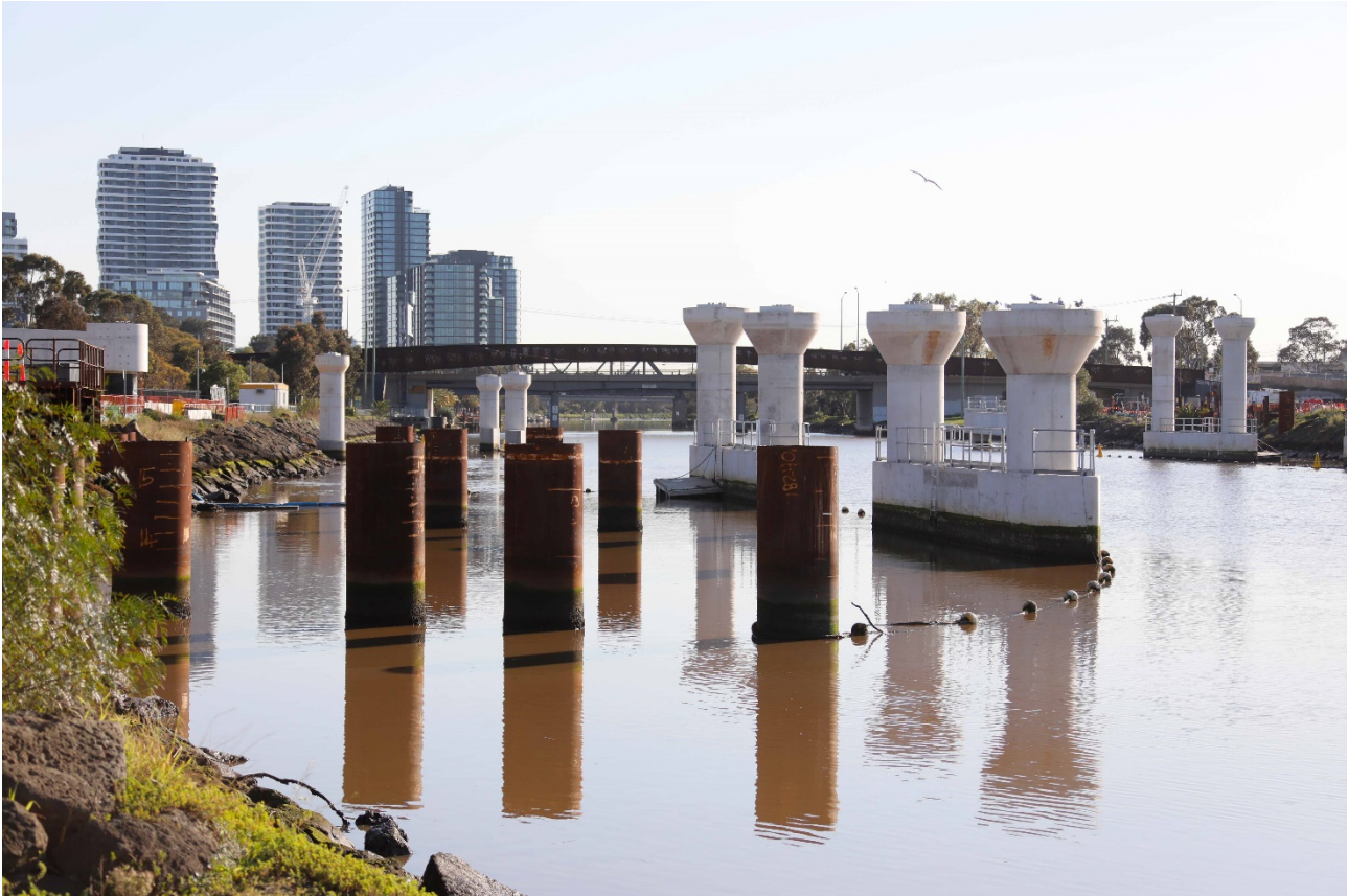
Photo 5 – Substructure works for bridges over Maribyrnong River – East Zone (Source: WGTP MTIA, 8 September 2021)
