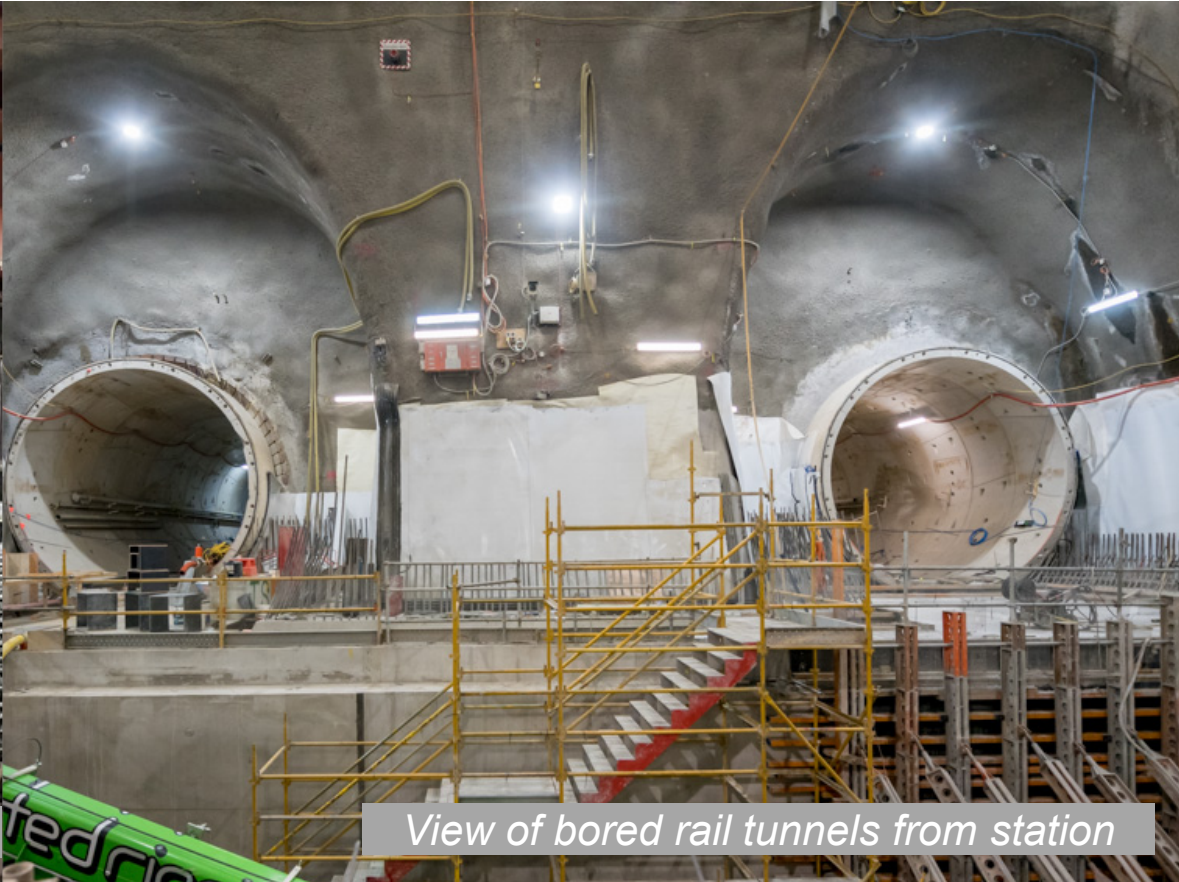
B4 slab poured at Franklin Street west
