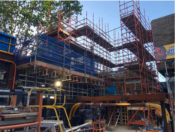
Temporary deck construction
