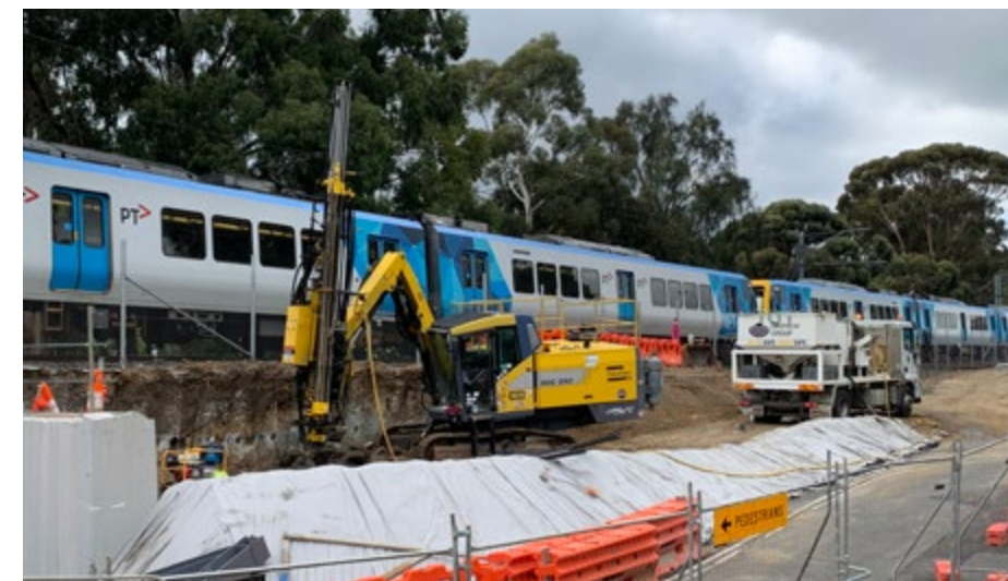
Works underway in Greensborough
