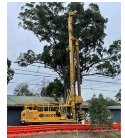
Piling rigs at work in Diamond Creek
