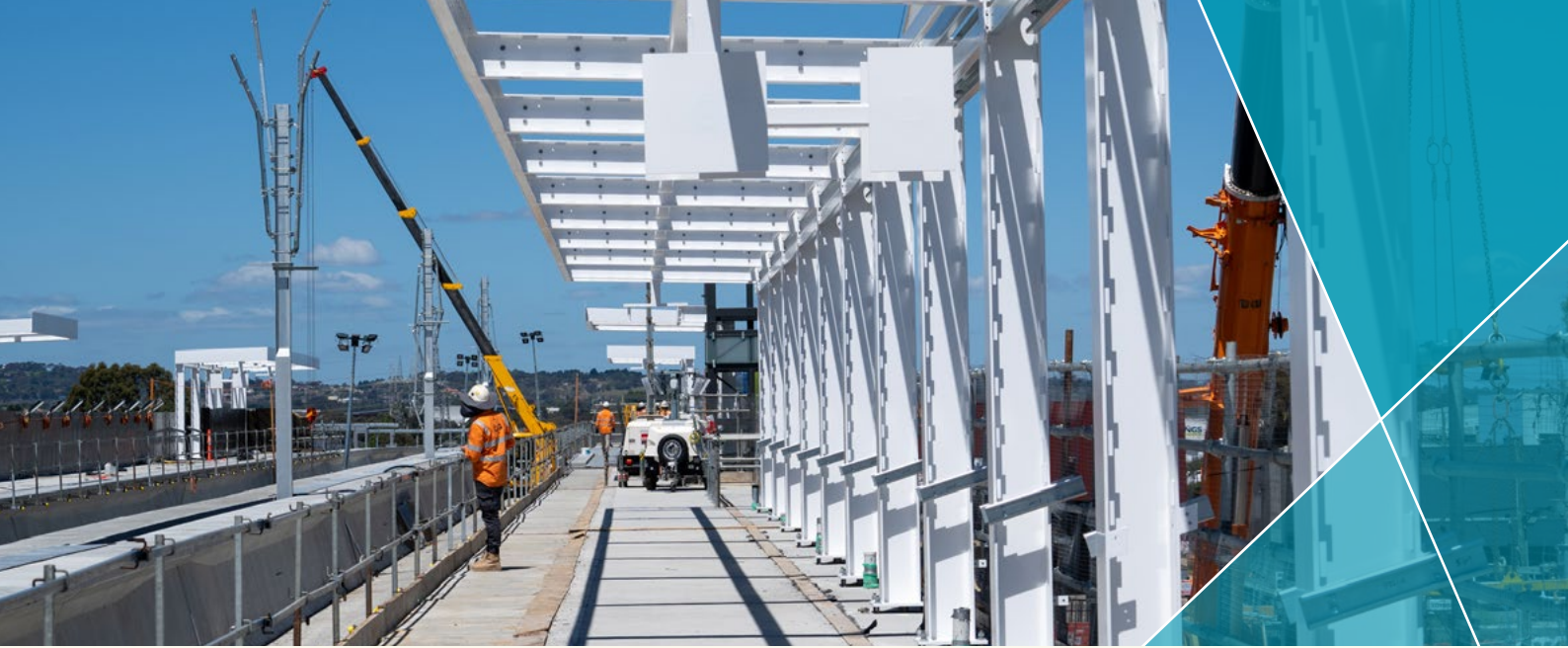
New canopies have been installed on the station platforms
