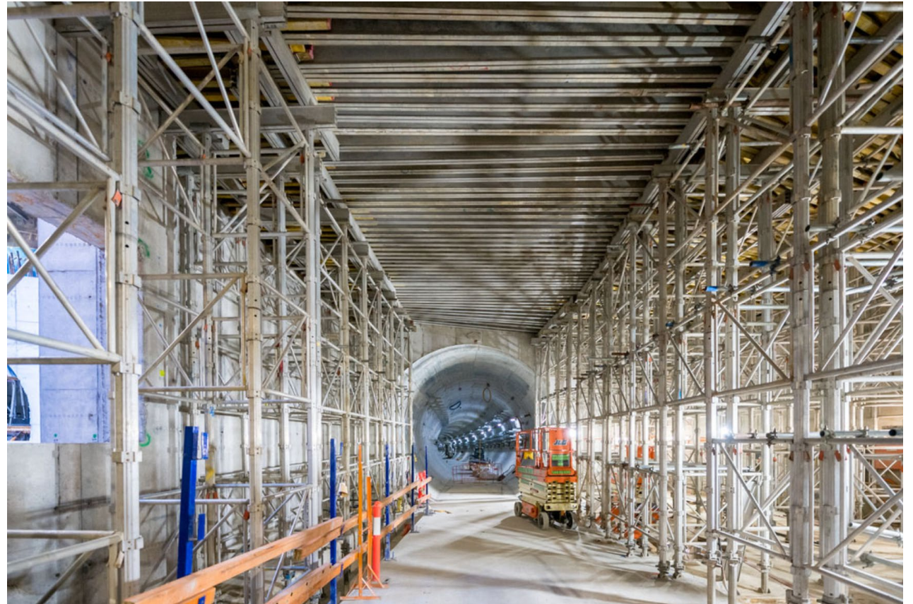
Falsework to support B1 slab construction
