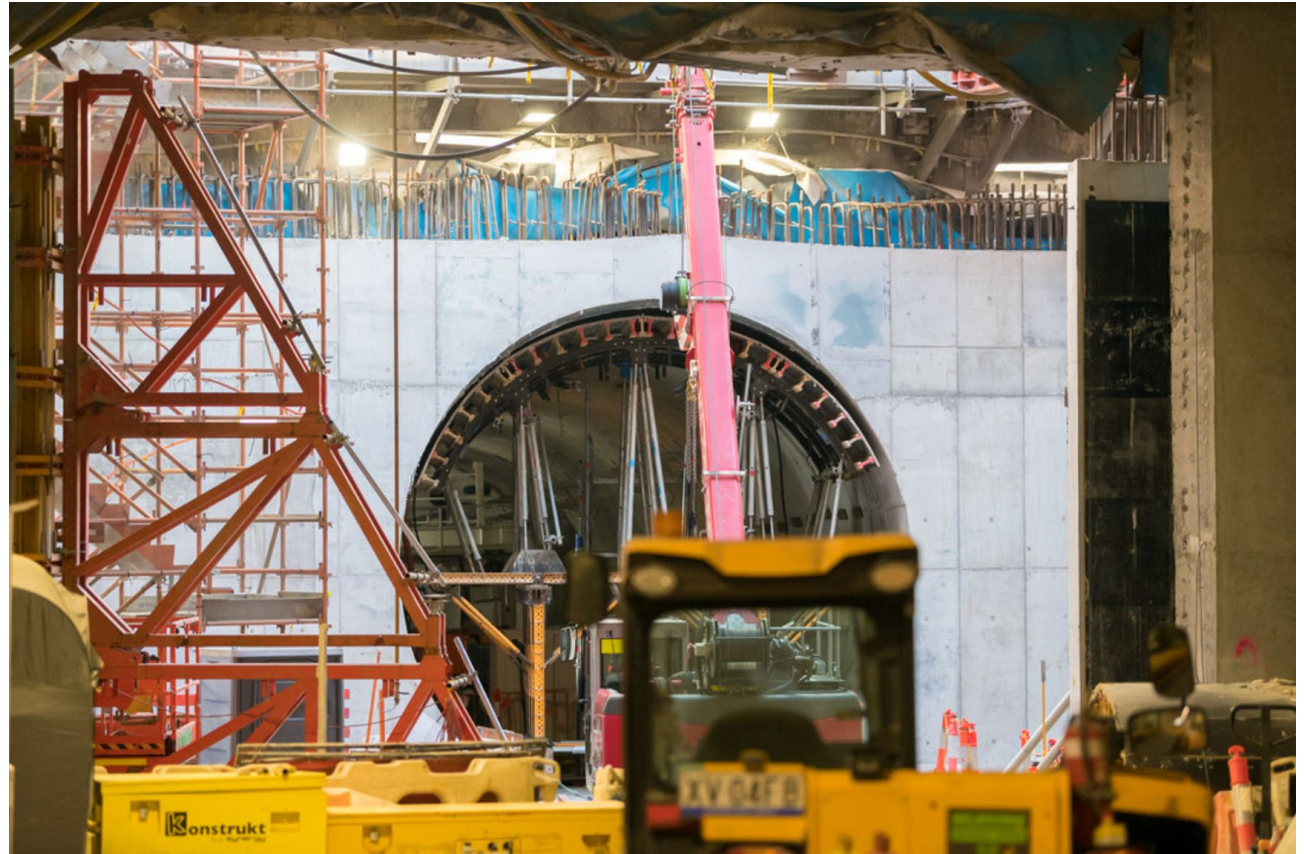
Finished westbound stub tunnel prior to formwork removal
