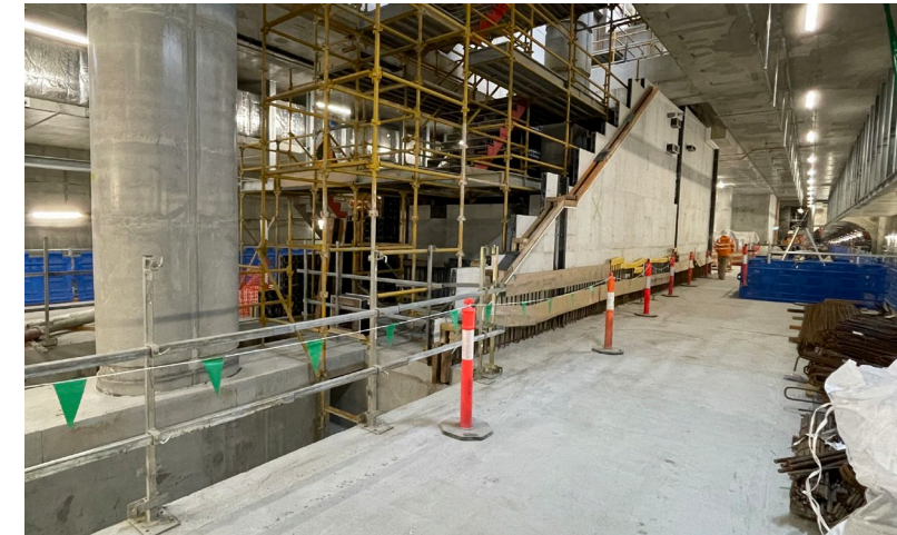
Platform level works
