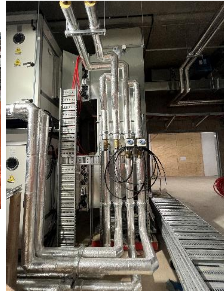
Plant rooms (concourse level)
