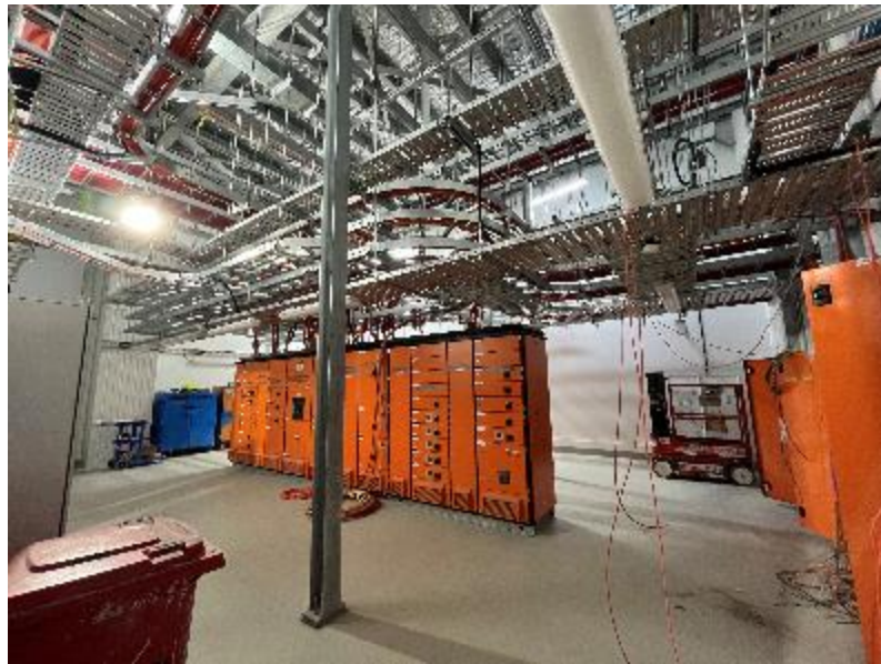
LV switch room fit out (concourse level)
