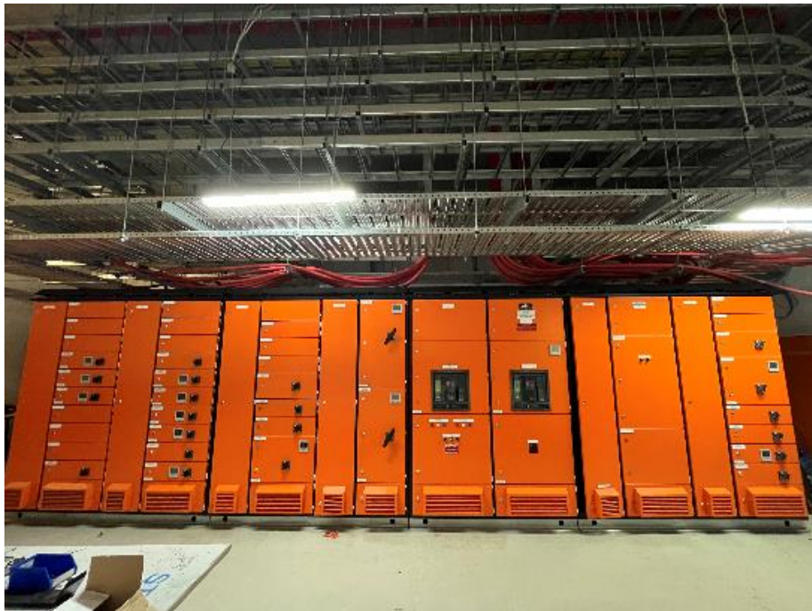
LV switch room fit out (concourse east)
