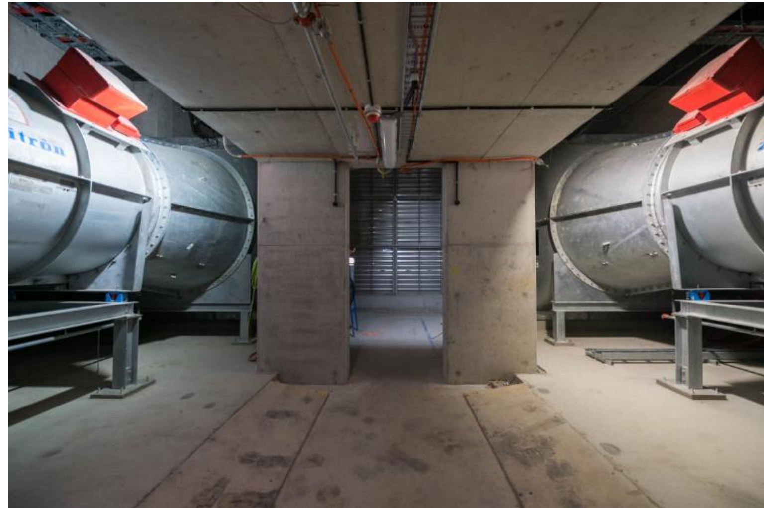
Over track exhaust (OTE) and tunnel ventilation fan rooms fit out
