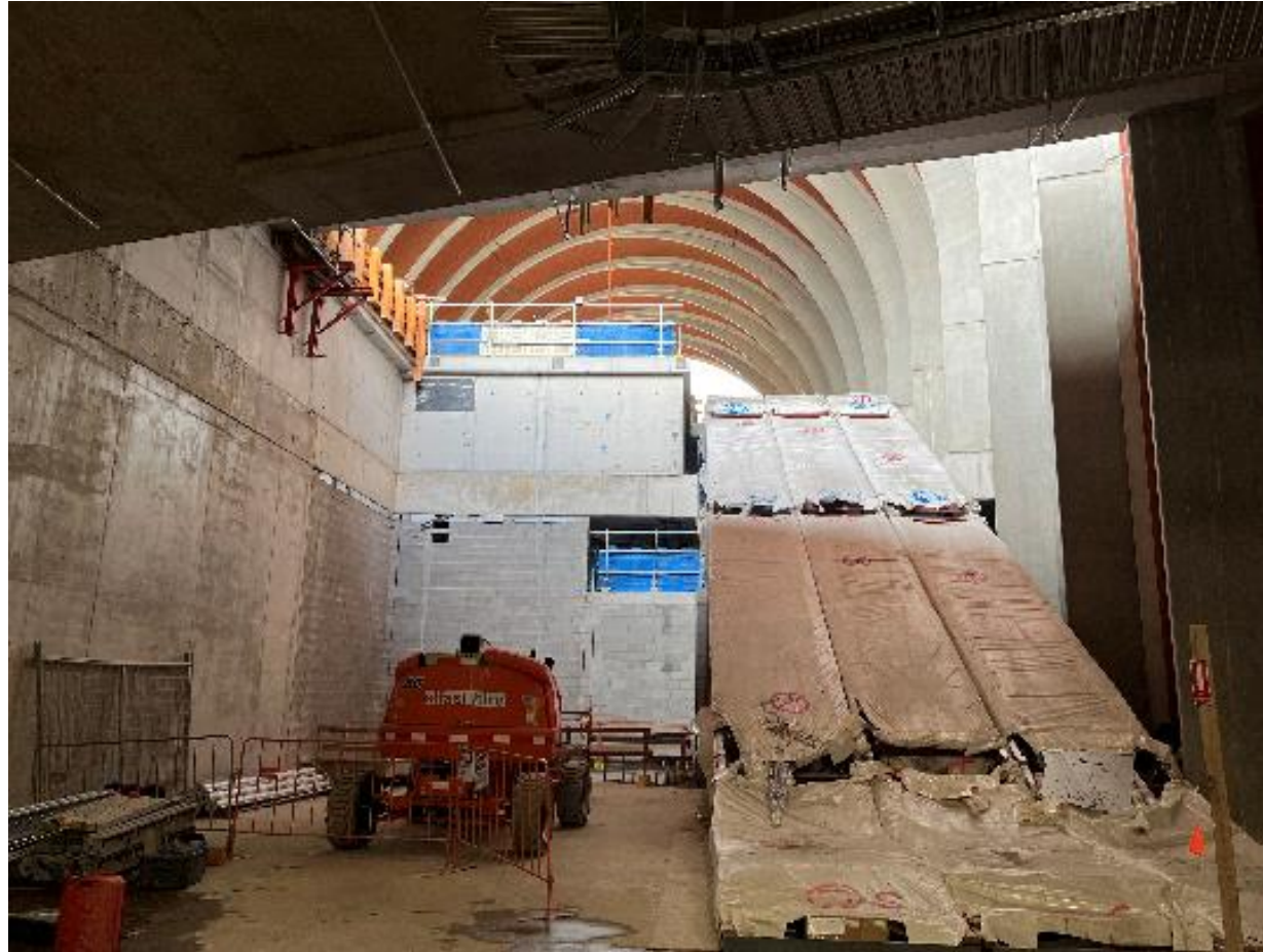
Escalators down to concourse level
