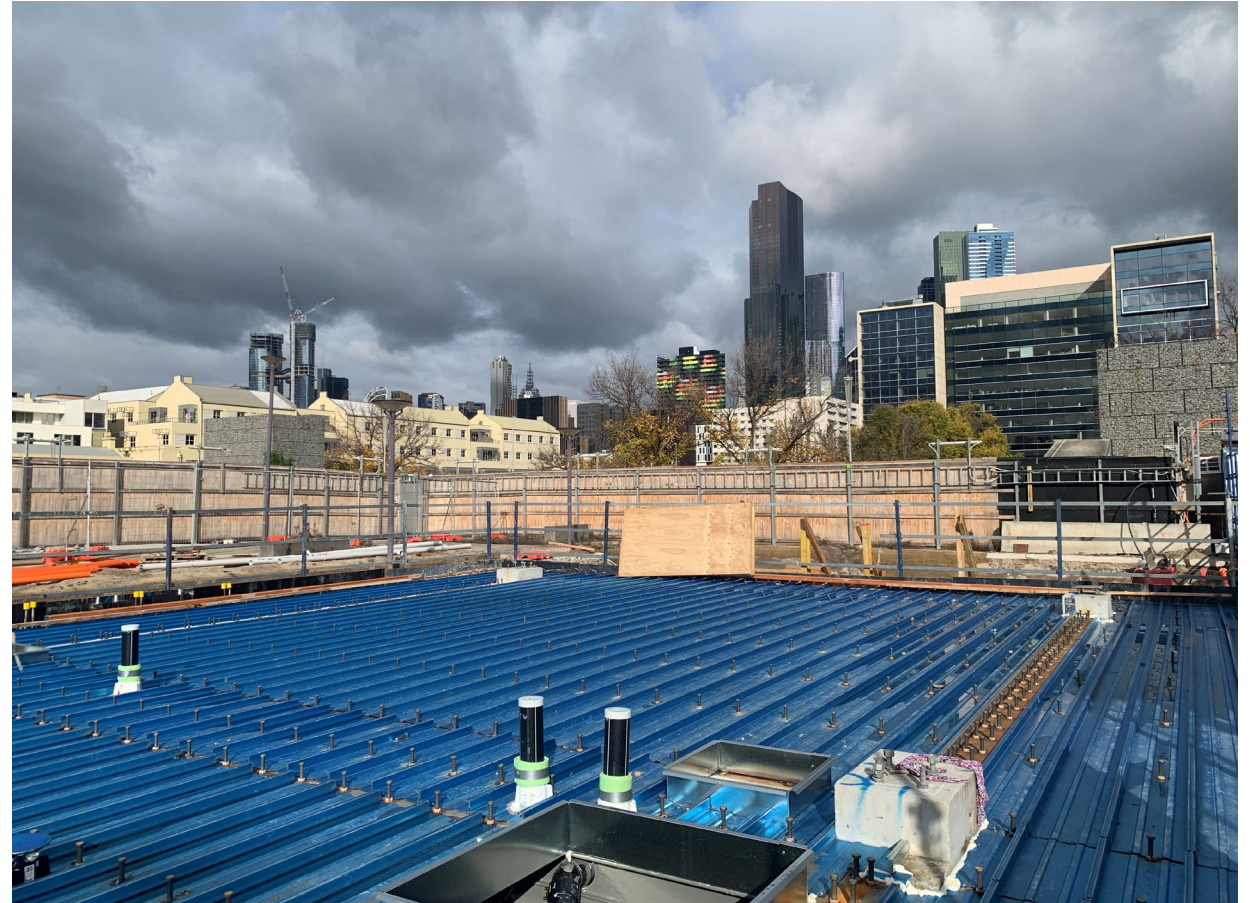
Chiller plant structural steel
