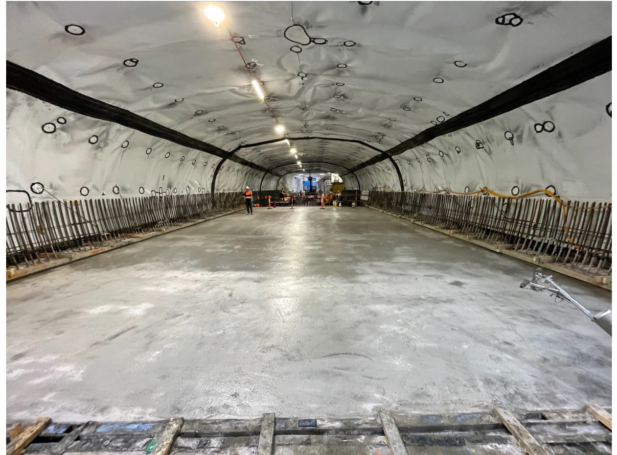
Royal Parade underpass base slab
