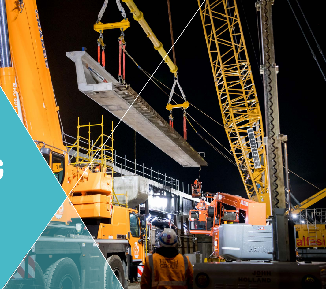
L-beam installation on the Reservoir Level Crossing Removal Project
