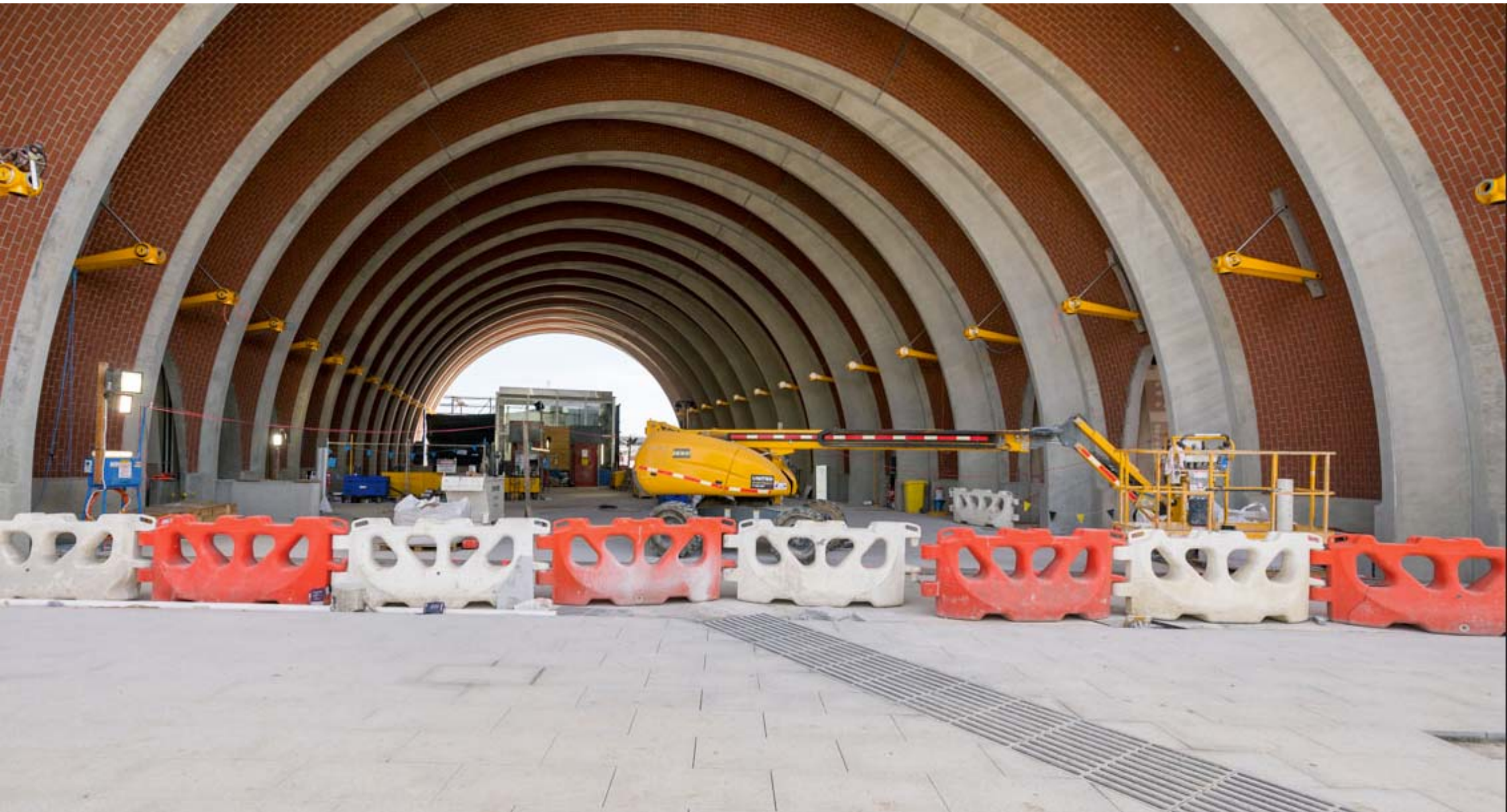
Station entrance tactiles and tiling installation
