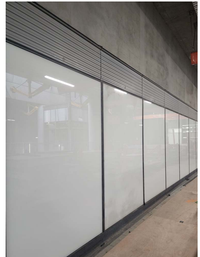
Colour back glass installation
