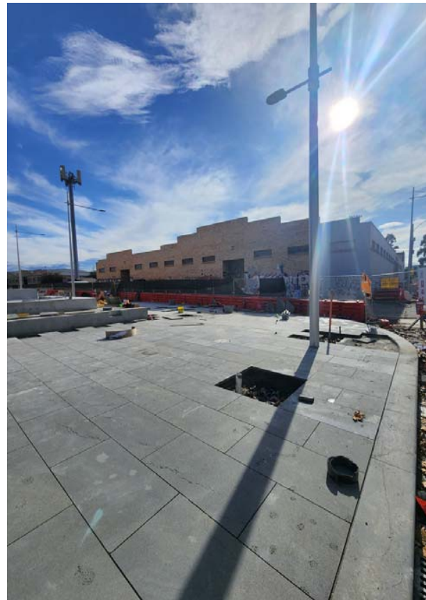
Laurens Street west - Kerbing and paving
