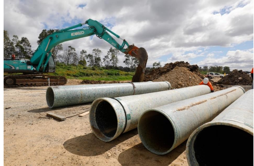
Recycled plastic pipes in action on a Victorian road project
